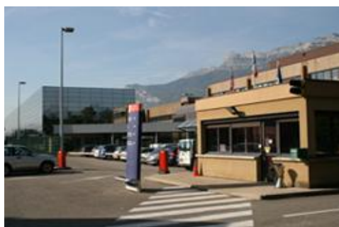
Figure 6: BD Pont de Claix site
