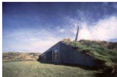
51 - Maison Marshall, Melbourne. Date NC, © Denton Corker Marshall
