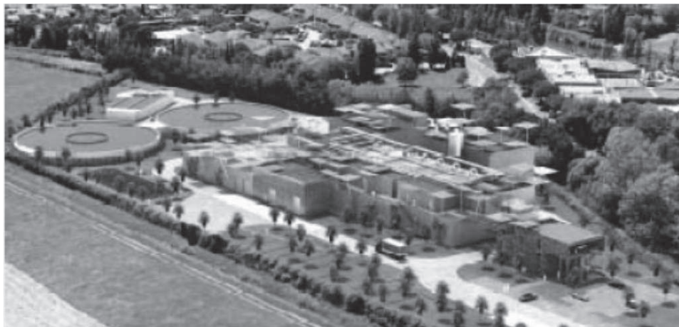
Figure 22 - Station d'épuration Aquaviva
