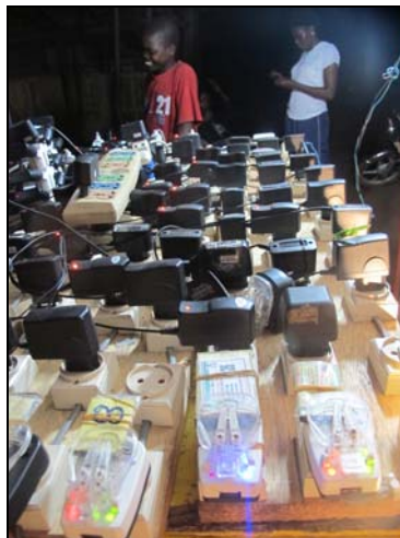
Charging station in a village in Bong Mines, Liberia (© Julie Thiery)
