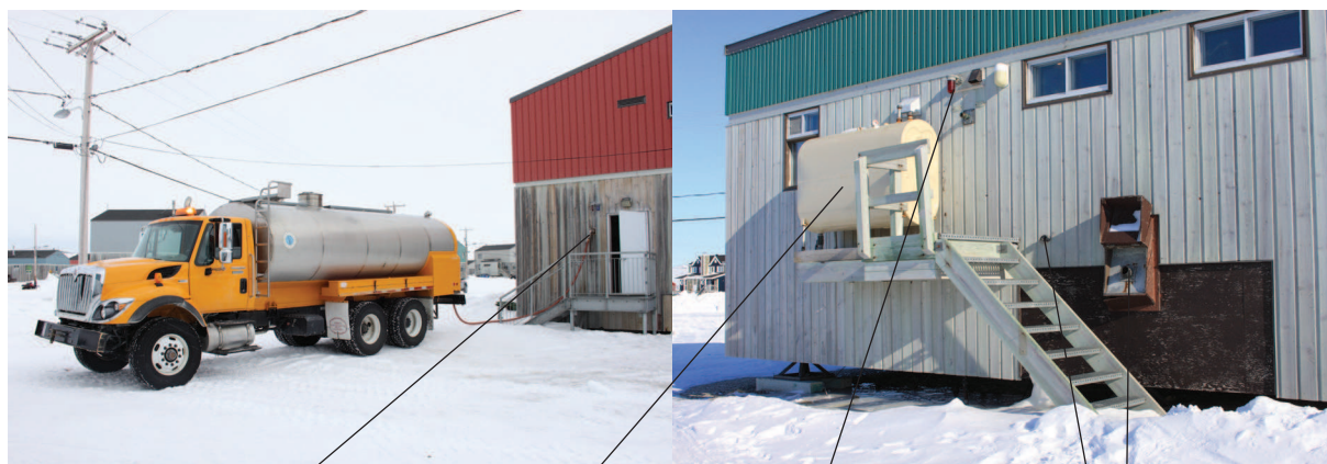
Alimentation eau potable
