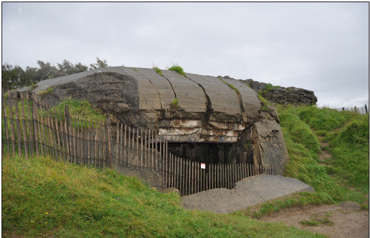
Figure 28 : Casemate H669 (photo A. Quereilhac).
