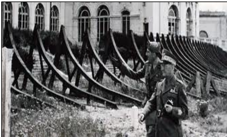
Figure 8: rail Curtoir (Source: musée- grand-bunker.com)
