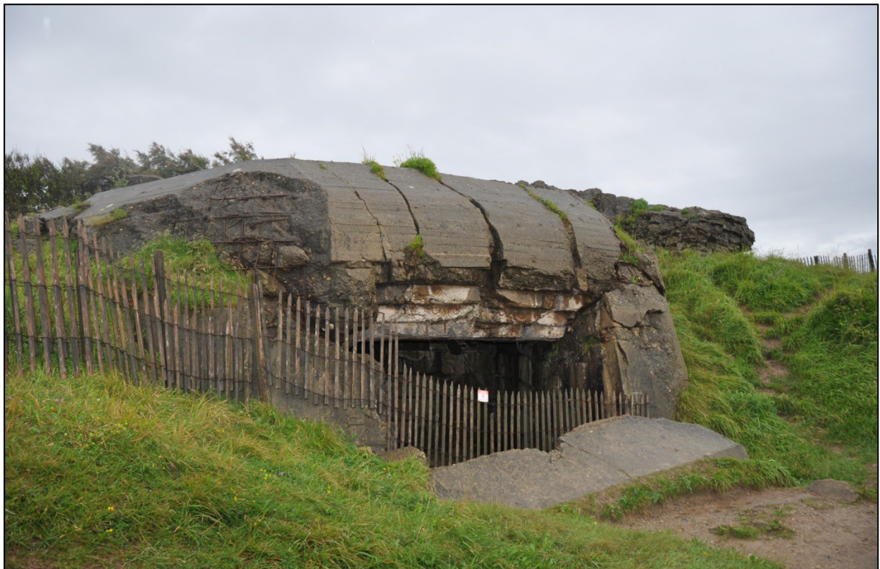
Figure 28 : Casemate H669 (photo A. Quereilhac).
