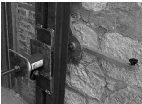
Fig. I.48 – Test d’arrachement, château Marchesale, San Giuliano di Puglia, Italie [ICC + 06]
