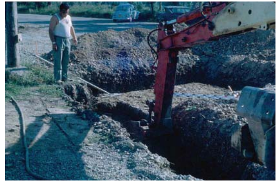
Figure 37 Chantier UPAT Source: Collection Image Jean-Henri, FABRE
