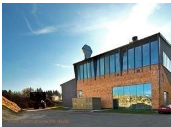
Figure 10. Zeltweg Power Station, Austria (industcards 2012)
