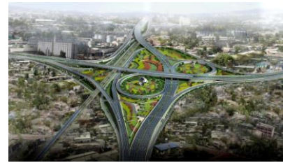
Figure 52 Gottera interchange Source : AUL
