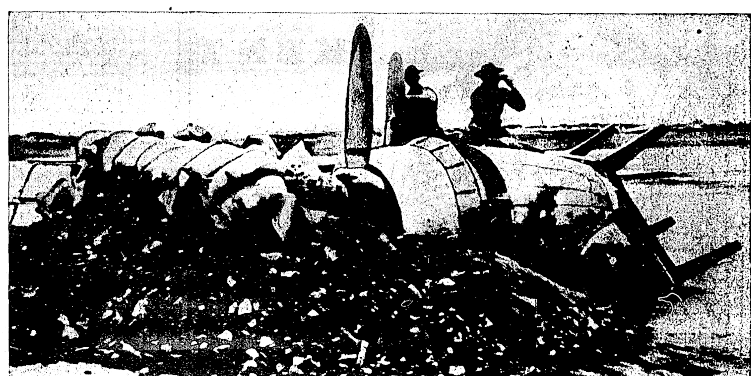
Using a part of a damaged plane, sandbags, and piled earth, soldiers at Hickam field improvised a machine gun nest during the Japanese bombing raid and were on the lookout for enemy planes.
