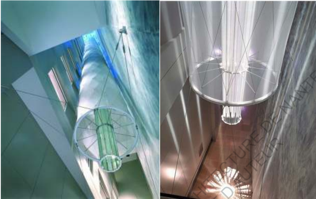
Figures 4-17 Photographie. Lumiduc prismatique. James Carpenter. Washington DC. USA ( carpenterlowings.com/portfolio_page/solar-light-pipe/ )
