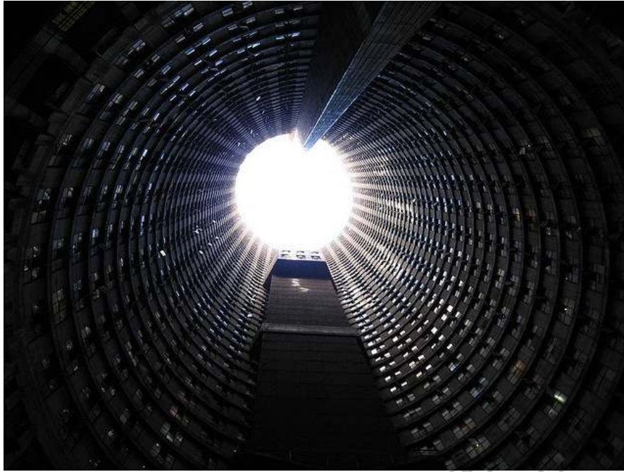
Figure 1-18 Photographie, Ponte Building, Johannesburg 12
