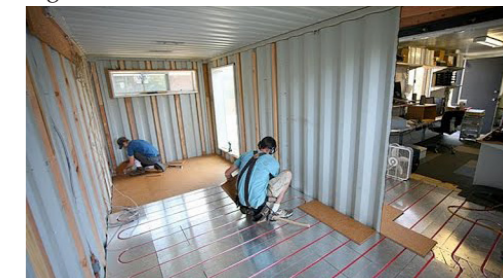
Fig.46: conteneur de construction.
