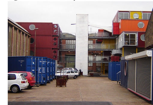
Fig.33: Circulations, Container City I et II.
