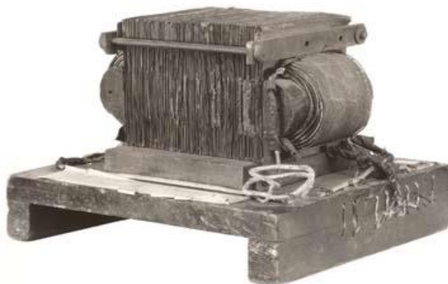
Fig.2. The first commercial electric transformer made by William Stanley
