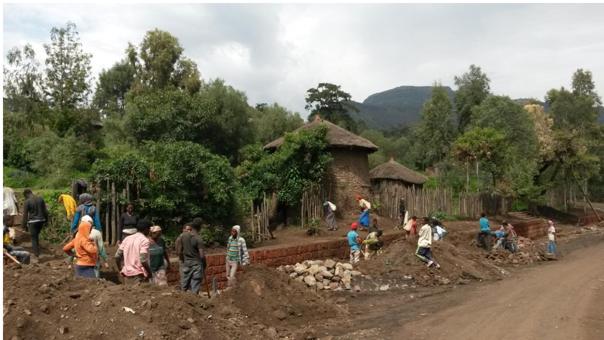
Fig. 3.3. Repaving the "Honey street"
