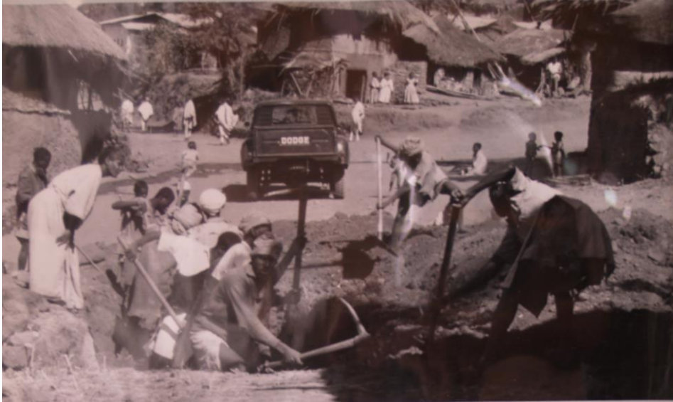
Fig.2.8. Angelini's workers digging the trenches
