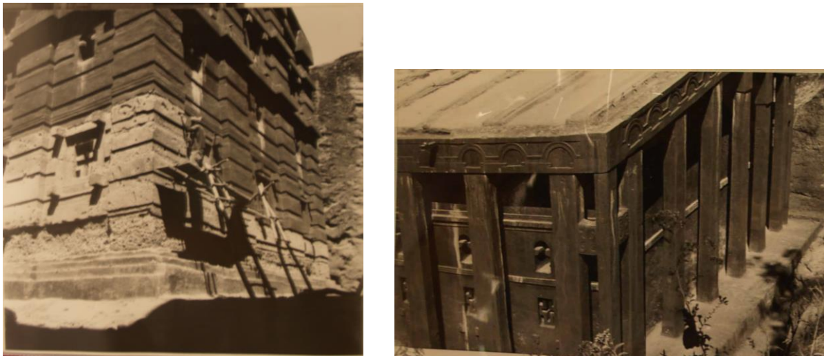
Fig. 2.5. Plastering and painting the walls of Bete Amanuel and Medhane Alem
