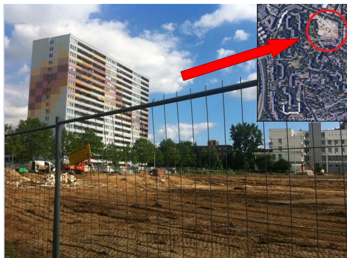
Figure 20: Construction started at the north-west side of Ben-Gurion -Ring.
