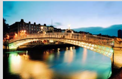
Fig. 67 - Ha'Penny Bridge, Dublin
