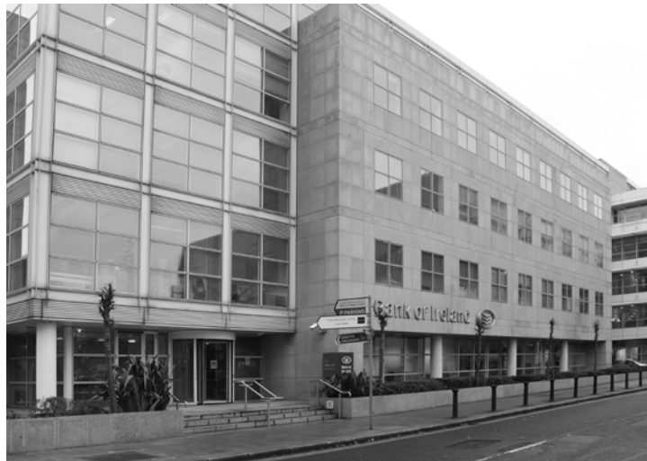
◀ Bank of Ireland, Mayor Street Upper, 2016
