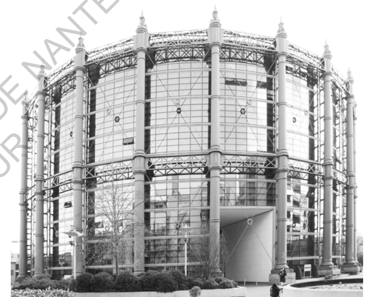
▶ Réhabilitation de silo de stockage. Gaswork housing par OMP architects, South Lotts Road
