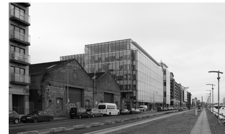
Immeubles de bureaux, Sir Rogerson's Quay, Grand Canal Docks
