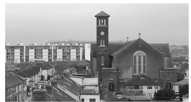
St Joseph's Catholic Church, Church Road (East Wall)
