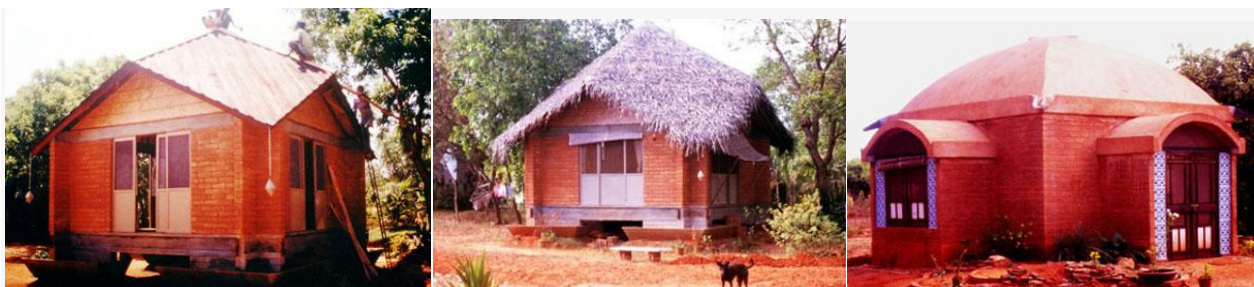
Figure 84 (Left) Legaum prototype with wooden shingles and interlocking CSEB. Source: (Auroville Earth Institute , Undated)
