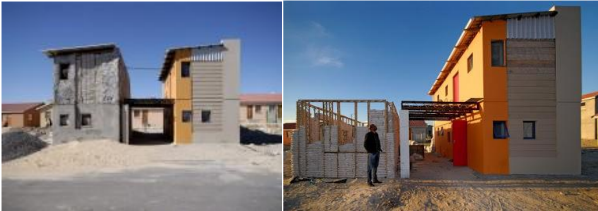
Figure 99 (Left&right) Sandbag in-fill method in the Mitchell's Plain project. Source: (designindaba, 2009)
