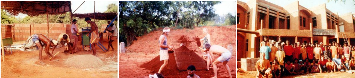
Figure 87 (Left & middle & right) Community participation: Block making and soil sieving. Source: (Auroville Earth Institute , Undated)
