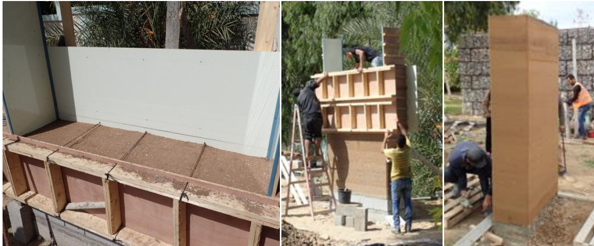
Figure 58 (Left, middle, & right) Rammed earth test walls in Gaza Strip. Source: (Paccoud, 2015)
