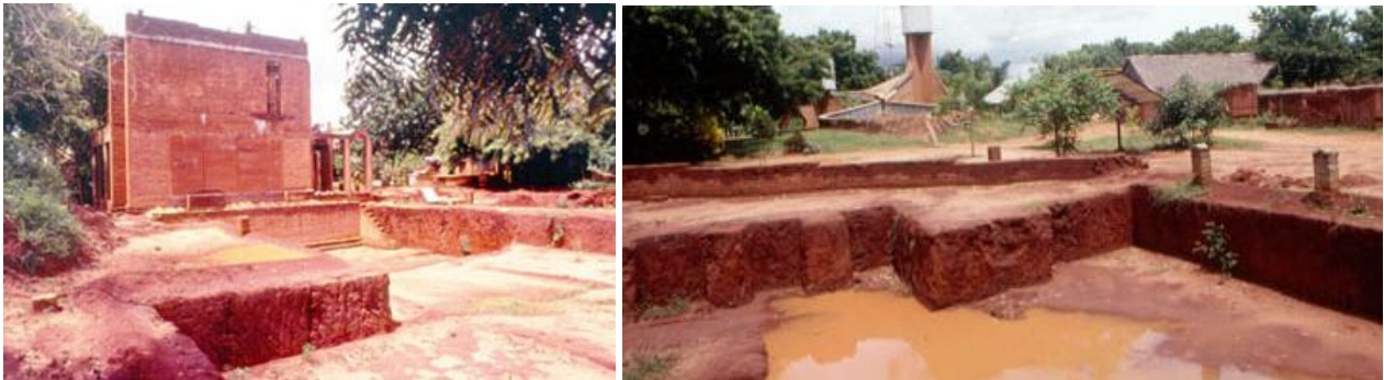
Figure 65 ( Left & Right) Excavation of the basement floor – 1.2 m below ground level. Source: (Auroville Earth Institute , Undated)
