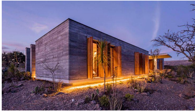
Figure 32 Casa Candelaria made of rammed earth in Mexico. Source: (Dezeen, 2016)
