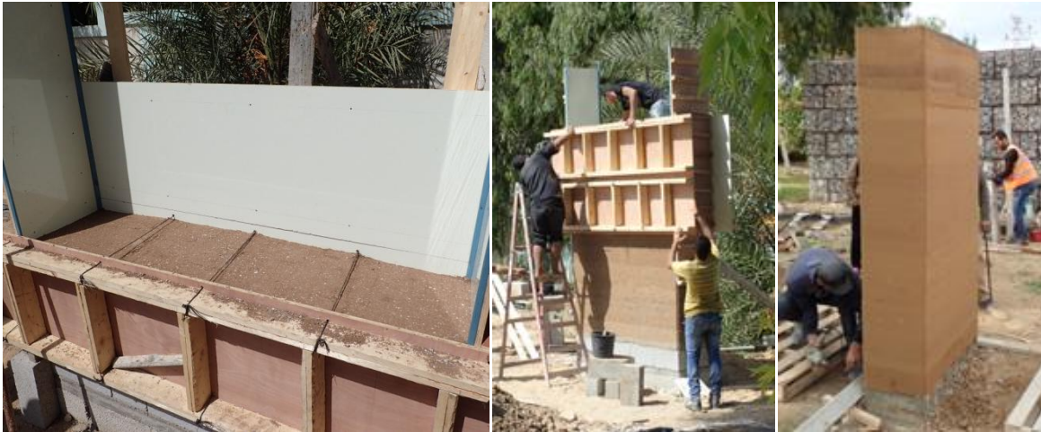
Figure 58 (Left, middle, & right) Rammed earth test walls in Gaza Strip. Source: (Paccoud, 2015)
