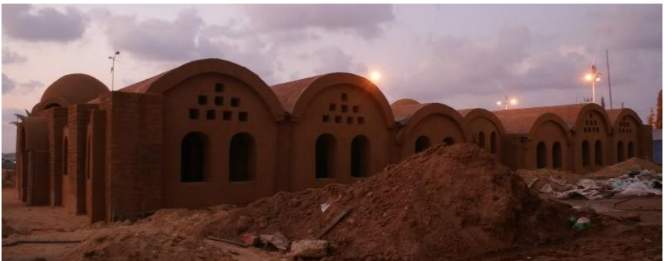
Figure 1 Governmental building using Mud-bricked in Gaza. Source: (Fayez, 2009)
