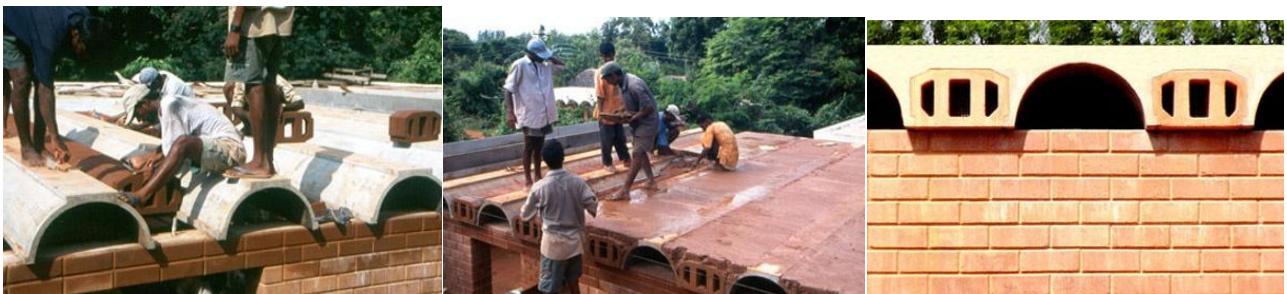
Figure 78 (Right) Floor with Hourdi blocks and ferrocement channels. Source: (Auroville Earth Institute , Undated)
