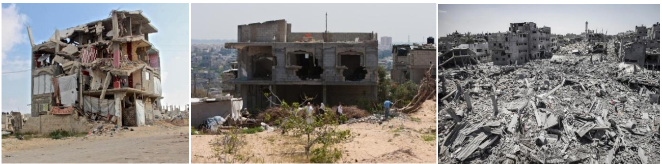
Figure 7 (left) Severe Damaged apartment, source: (Harriet, 2015)
