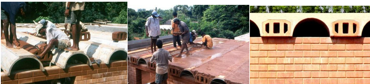
Figure 78 (Right) Floor with Hourdi blocks and ferrocement channels. Source: (Auroville Earth Institute , Undated)
