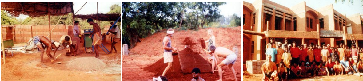
Figure 87 (Left & middle & right) Community participation: Block making and soil sieving. Source: (Auroville Earth Institute , Undated)
