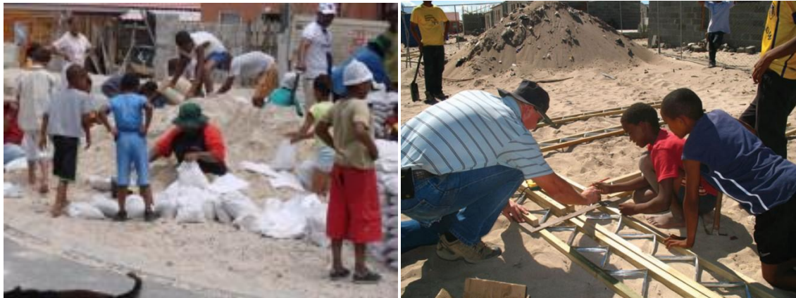
Figure 100 (Left) The community involvement in the building process. Source: (Smithsonian, 2011)
