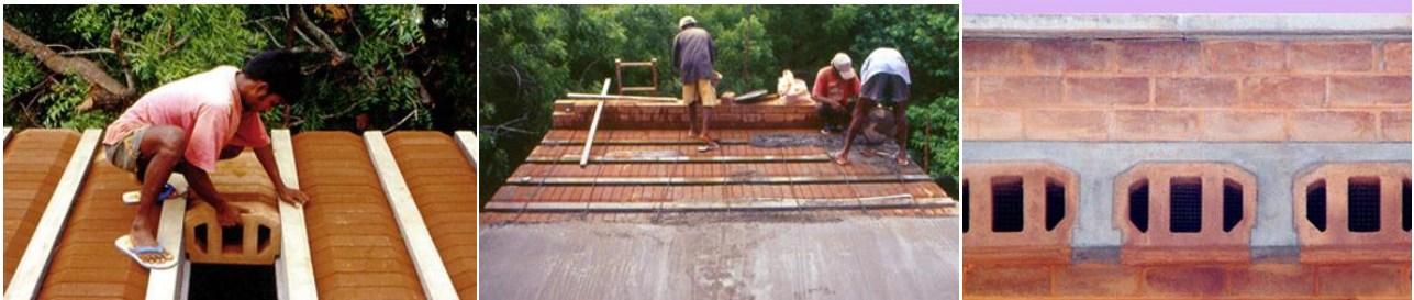
Figure 75 (Left) Adjusting Hourdi blocks on T beams. Source: (Auroville Earth Institute , Undated)
