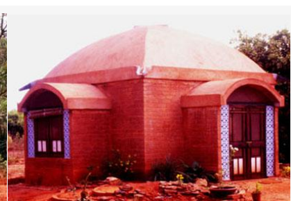
Figure 84 (Left) Legaum prototype with wooden shingles and interlocking CSEB. Source: (Auroville Earth Institute , Undated)
