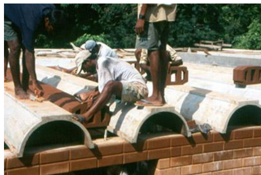
Figure 107 (Left) Hourdi blocks on reinforced concrete T beams. Source: (ballutblocks, Undated)
