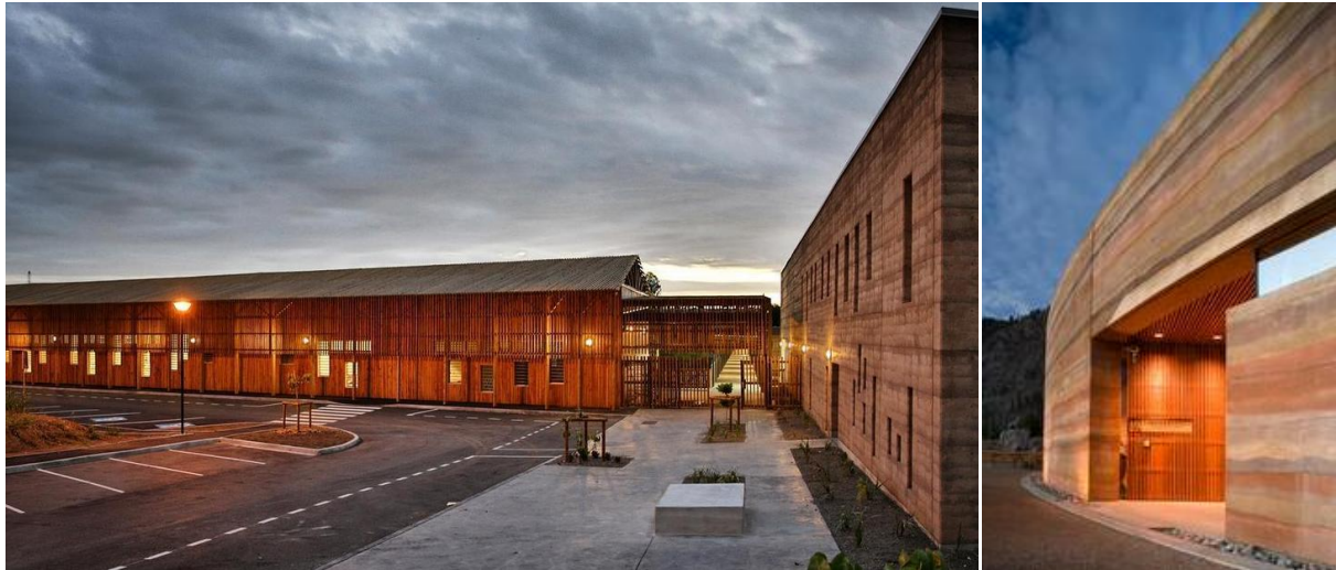
Figure 59 (Left) College Paiamboué facades made of rammed earth. Source: (CTB, 2016)
