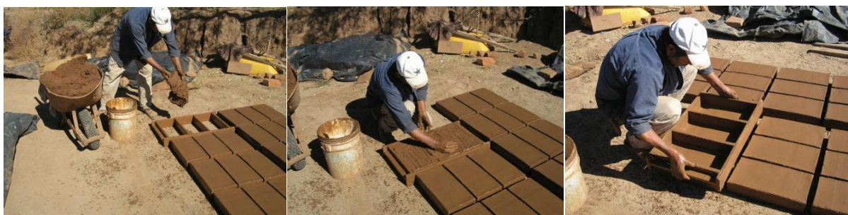
Figure 49 Adobe bricks production process. Source: (Sasabe Adobe, Undated)
