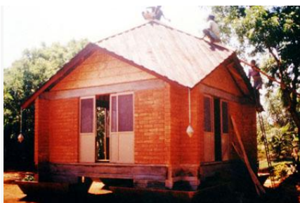
Figure 84 (Left) Legaum prototype with wooden shingles and interlocking CSEB. Source: (Auroville Earth Institute , Undated)
