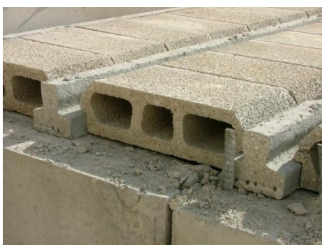
Figure 107 (Left) Hourdi blocks on reinforced concrete T beams. Source: (ballutblocks, Undated)
