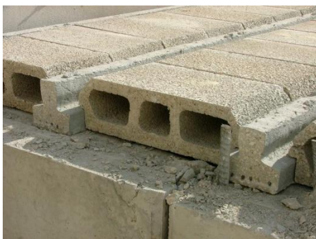
Figure 107 (Left) Hourdi blocks on reinforced concrete T beams. Source: (ballutblocks, Undated)
