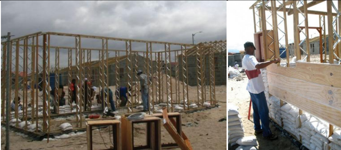
Figure 97 (Left) The structural framework (Eco-Beam). Source: (Duarte, 2008)
