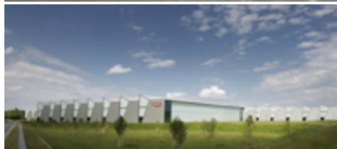
**18.** « For Kaufbeuren, other architects proposed a timber façade in their competition design. They were evidently not aware that the vapours emanating from the machine lubricants can dissolve the adhesives used in glued members. » **Details, « Industriebau », n°3, 2015, p160.**
