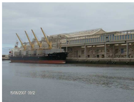
Figure 14 : Le terminal OCP.
