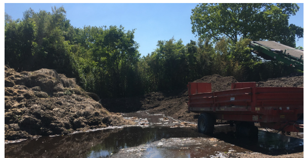
Figure 30: Stagnation des lixiviats (LOUVEAU, 2017)
