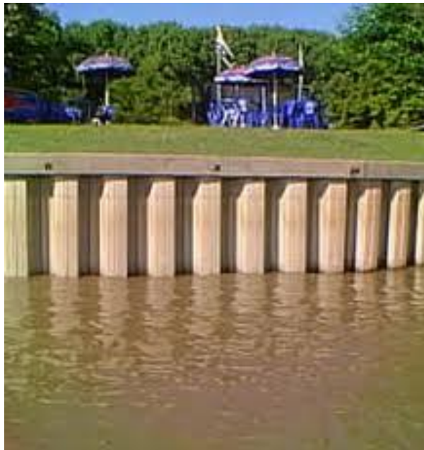
Figura 14: Tablestacas ( www.mdstrading.com.ar )
