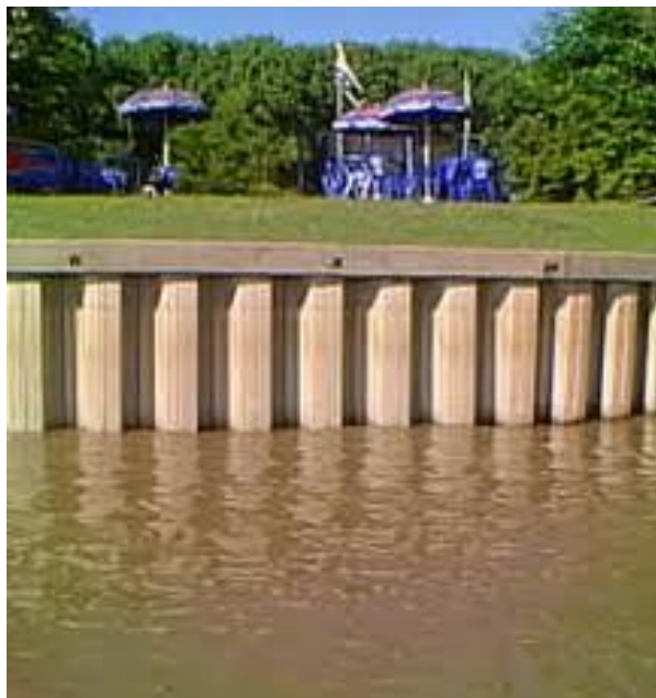
Figura 14: Tablestacas ( www.mdstrading.com.ar )
