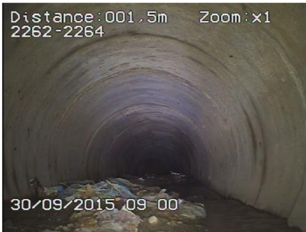
Figure 35 : Photo N°2262_0760 issues des inspections hydrozoom
