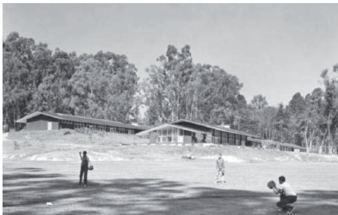
North Hillsborough School, E.Kump, 1955, façades Sud-Ouest, Modern Schools: A Century of Design for Education , R.Thomas. Hille, 2011
