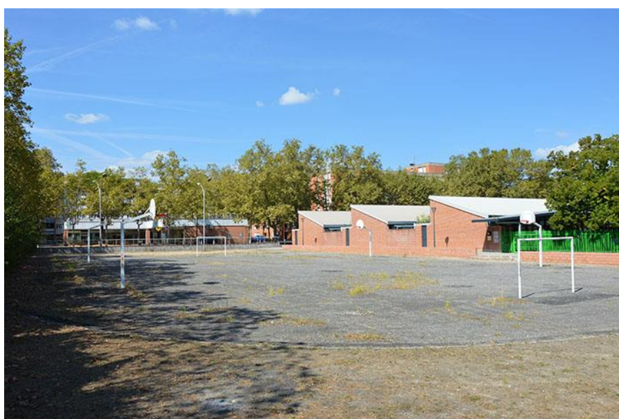
Figure 2 - Square Augereau, quartier Cantepau, Albi (81)
