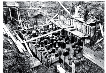
Wooden pylons sustain the soil in Venice. Above: the "Pylon Inserting Machine" is depicted in Giannantonio Rusconi's engraving ( On Architecture , 1590). Below: a picture showing pylon density required to support the weight of a building.
