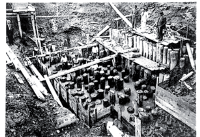
Wooden pylons sustain the soil in Venice. Above: the "Pylon Inserting Machine" is depicted in Giannantonio Rusconi's engraving ( On Architecture , 1590). Below: a picture showing pylon density required to support the weight of a building.
