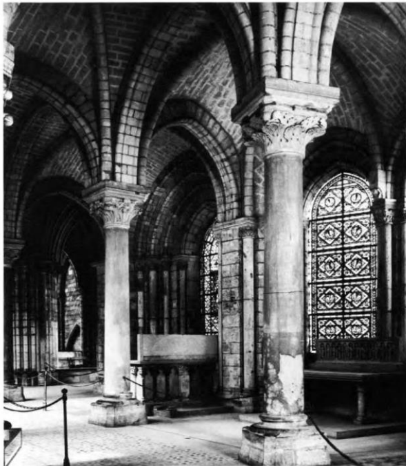
Fig. 10. Saint-Denis, ambulatory columns
