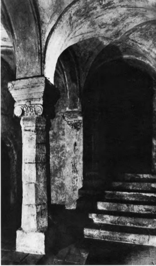
Fig. 15. Auxerre, Saint-Germain, crypt, octagonal column on south side
