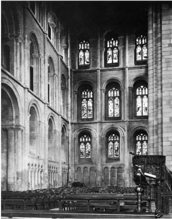
Fig. 1. Peterborough Cathedral, interior of north transept
