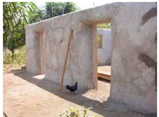
Figure 75- Murs finis (Source : Norman Padilla, ADIC)
