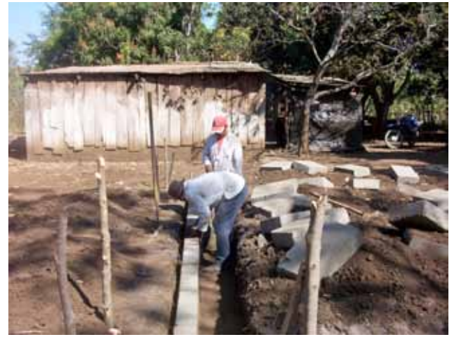
Figure 71- Pose des fondations (Source : Norman Padilla, ADIC)
