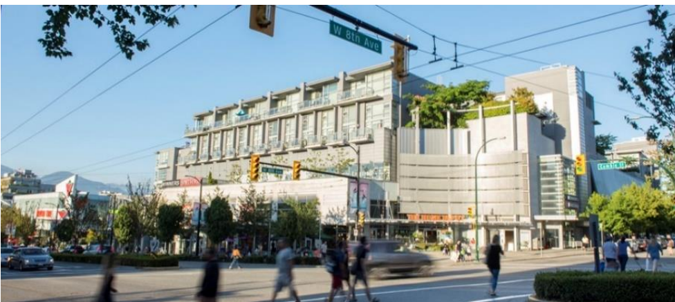
Figure 30 Façade de The Rise
