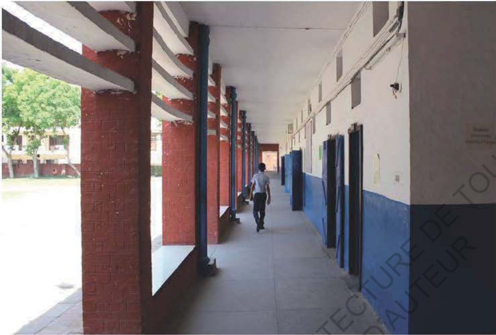
[134.] Coursive - Photographie de la Secondary School - S16.
