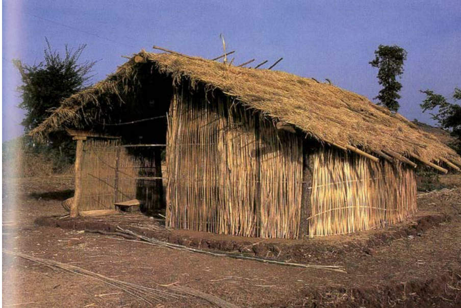
[8.] «A bamboo paddy thatched house. Eastern Gujarat», photographie issue du Traditional Buildings of India , p. 39.
