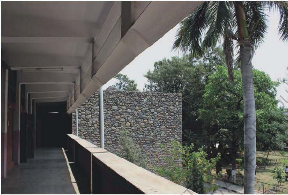
[137.] Coursive - Photographie de la Secondary School - S22.
