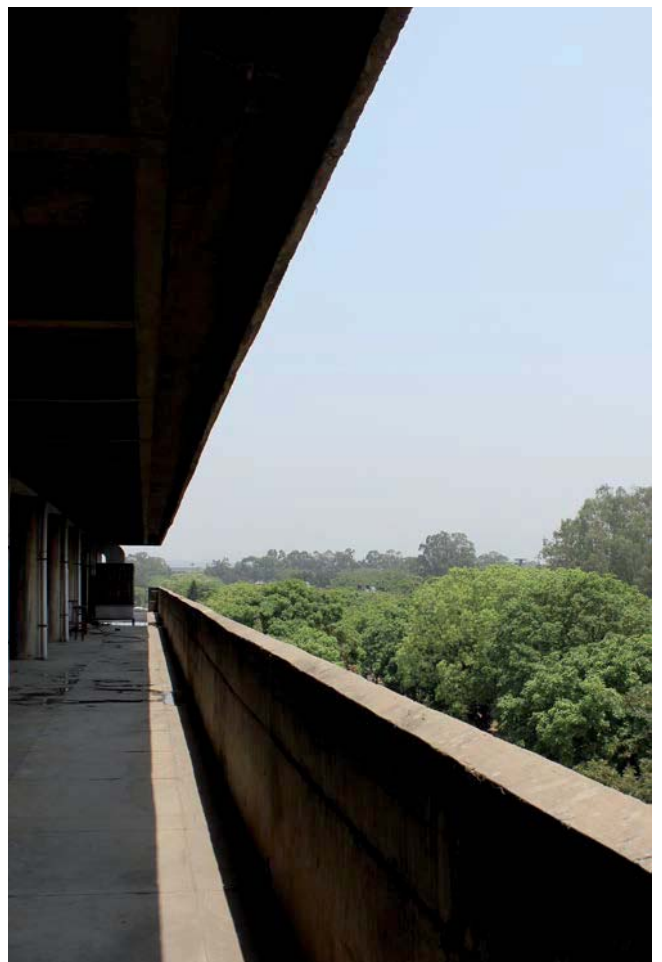
[118.] Galerie - Administration Building - S17.
