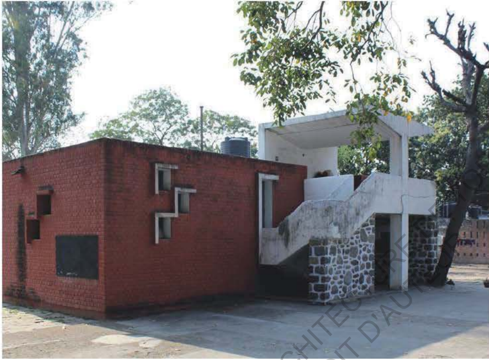
[170.] Toit-parasol / barsati - Photographie de la Nursery School - S23.
