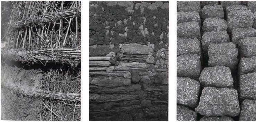
[28.] "Constructing the wall of a Rajasthani jhonpri or hut", photographie issue de Traditional Buildings of India , p.23.
