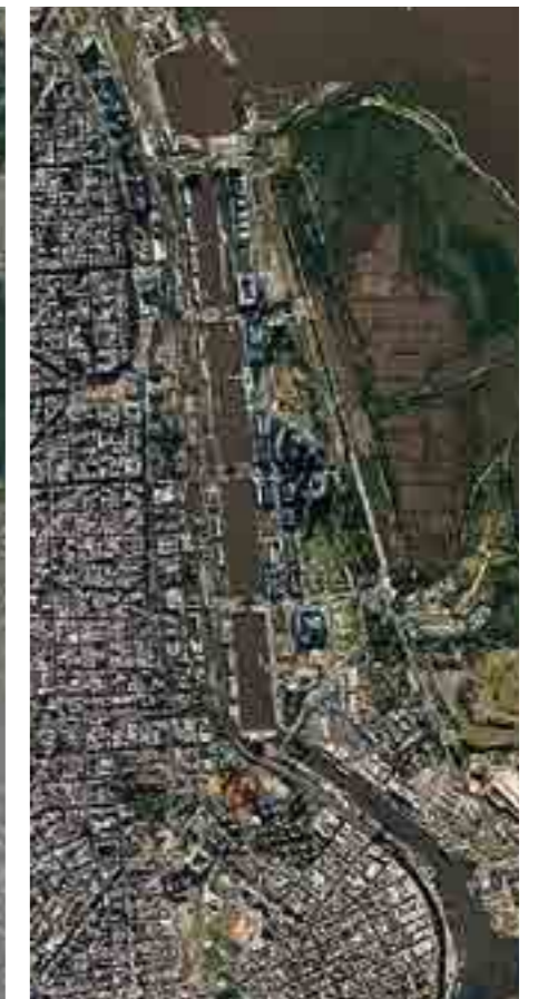
Figure 3. Port de Puerto Madero (Argentine) Source : Google Maps
