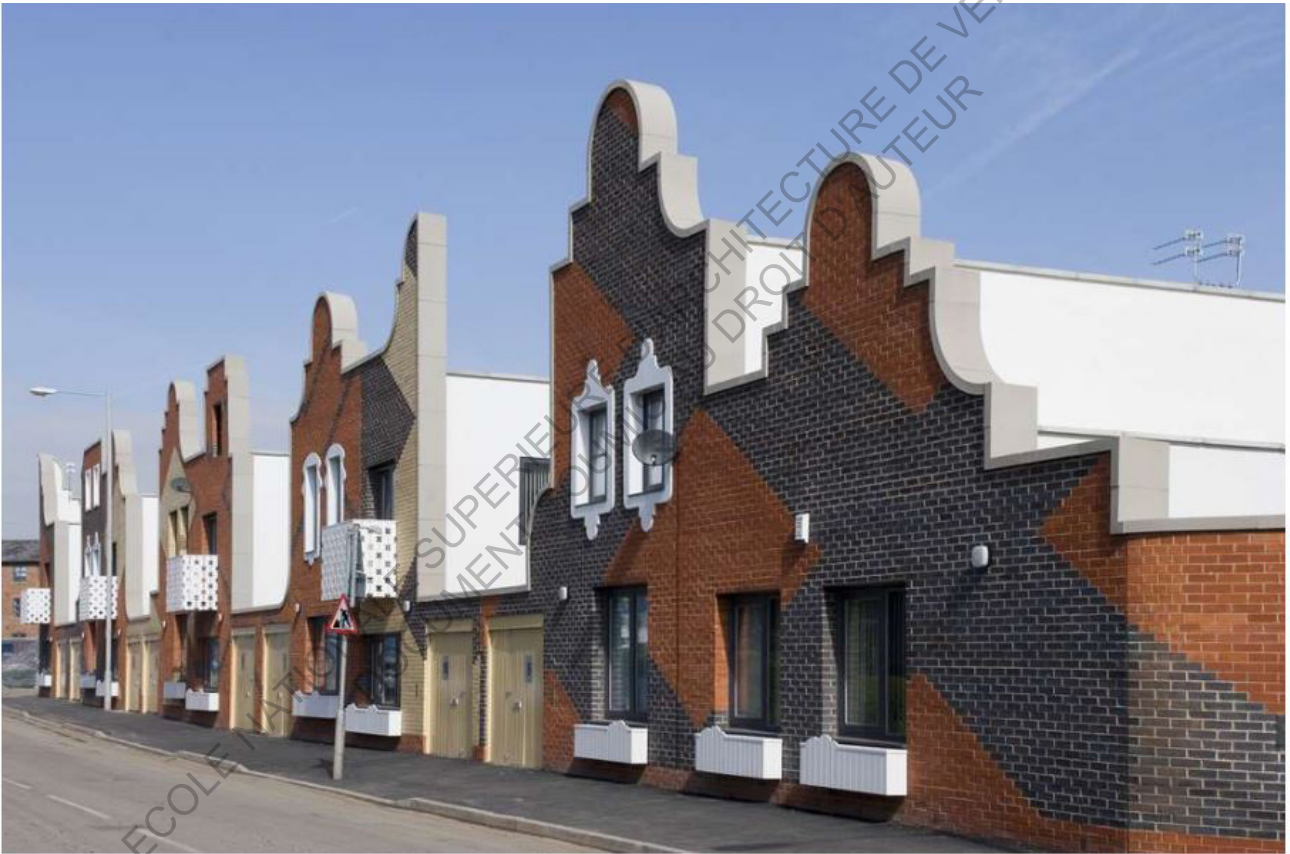
fig. 25 - Islington square social housing, New Islington (Manchester) FAT Architecture et Urban Splash 2006
