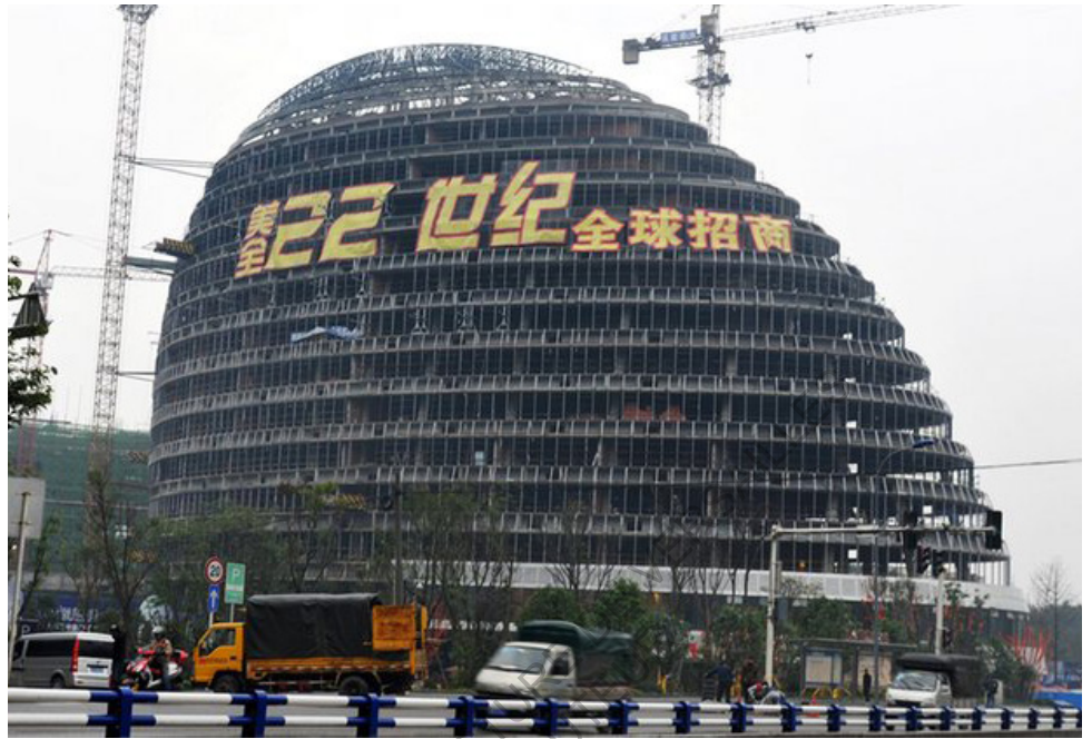
fig. 19 - The Meiqian 22nd Century Building , Chongqing
