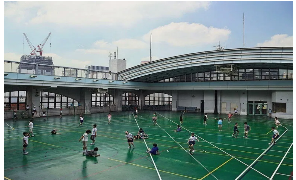
Shohei Elementary School, Tokyo
