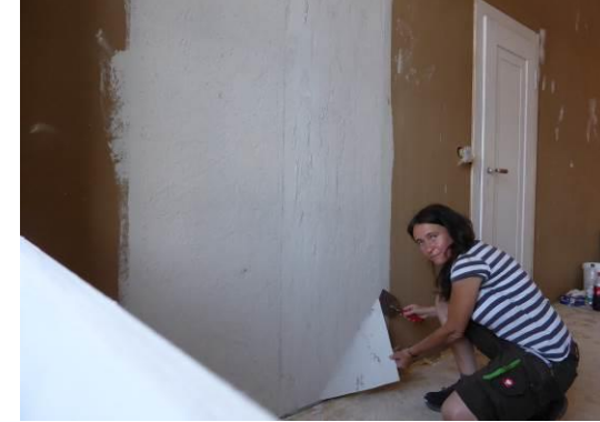
Removing wallpaper from wall because base colour did not show though the holes in the design as desired
