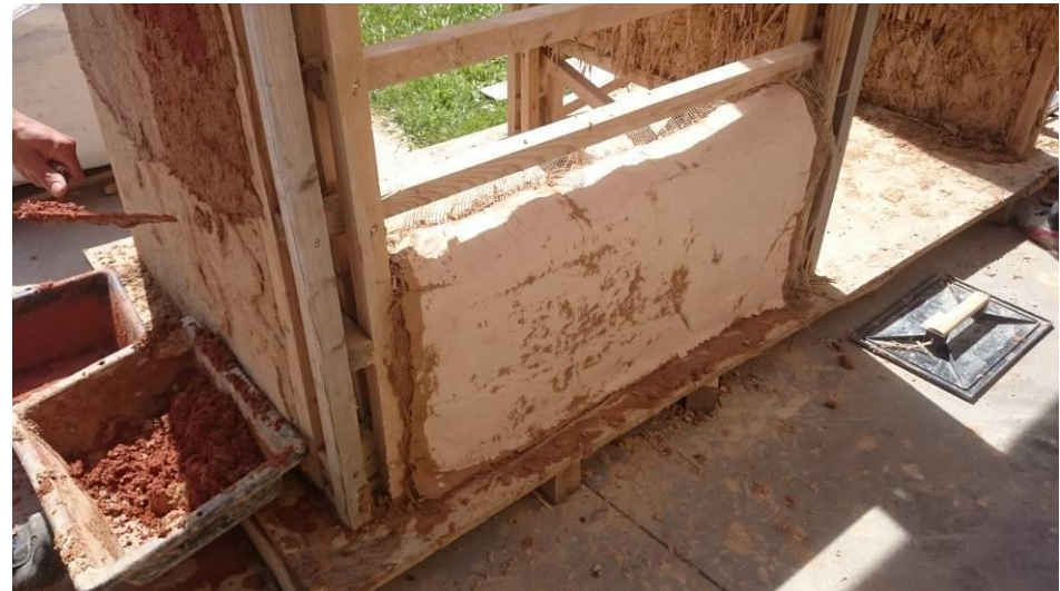
Clay wallpaper sample applied to lumpy straw clay infill wall at Grains d'Isère 2017
