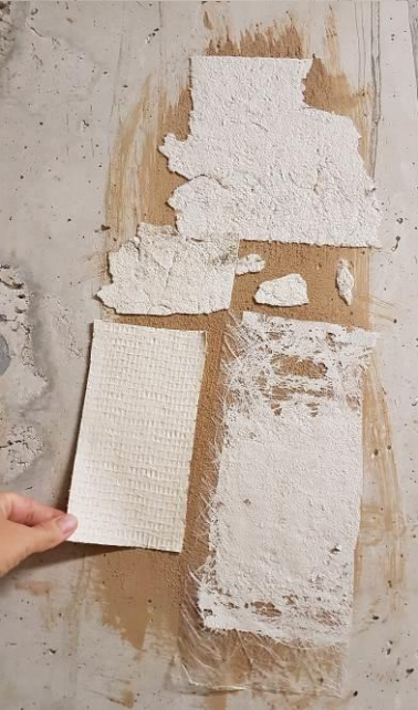
Various samples being removed from concrete substrate
