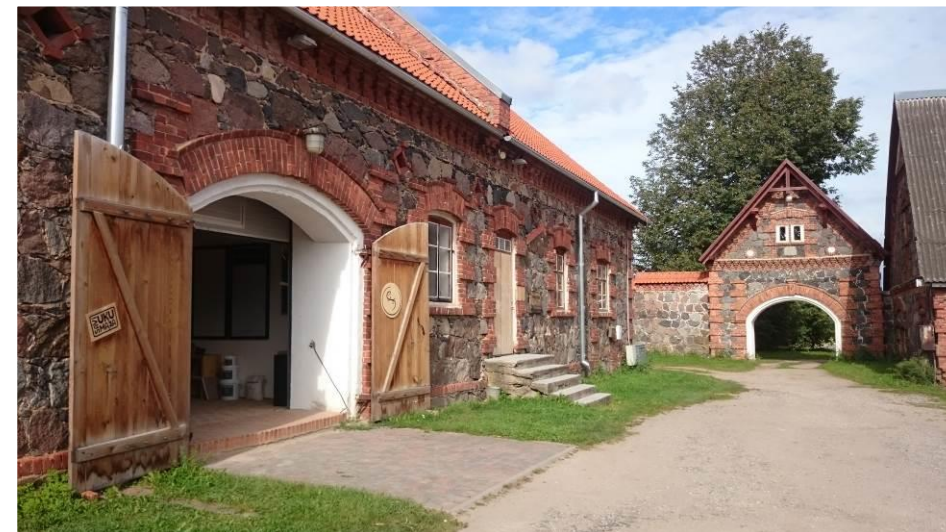
Saviukumaja Workshop and Showrooms at Mooste Manor, Estonia
