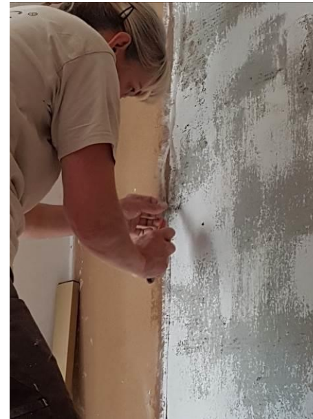
Above (left to right): series of pictures showing the mounting of the paper by the professional painter and decorator of Claytec using edge rolls, metal edge and carpet knife.
