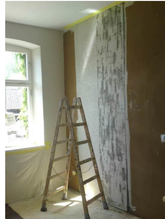
The very same piece of wallpaper stuck to a new umbra paint base
