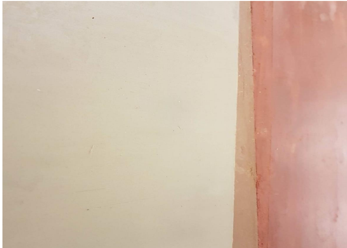
My own attempt at making and applying Hikitsuchi, a cellulose enforced clay finish
