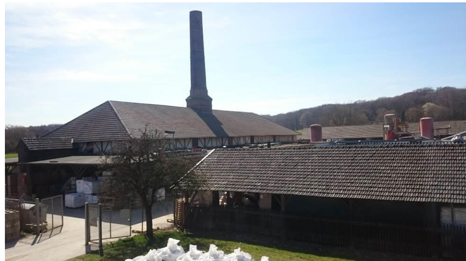
Storage, mixing and sales area at Claytec, 2018
