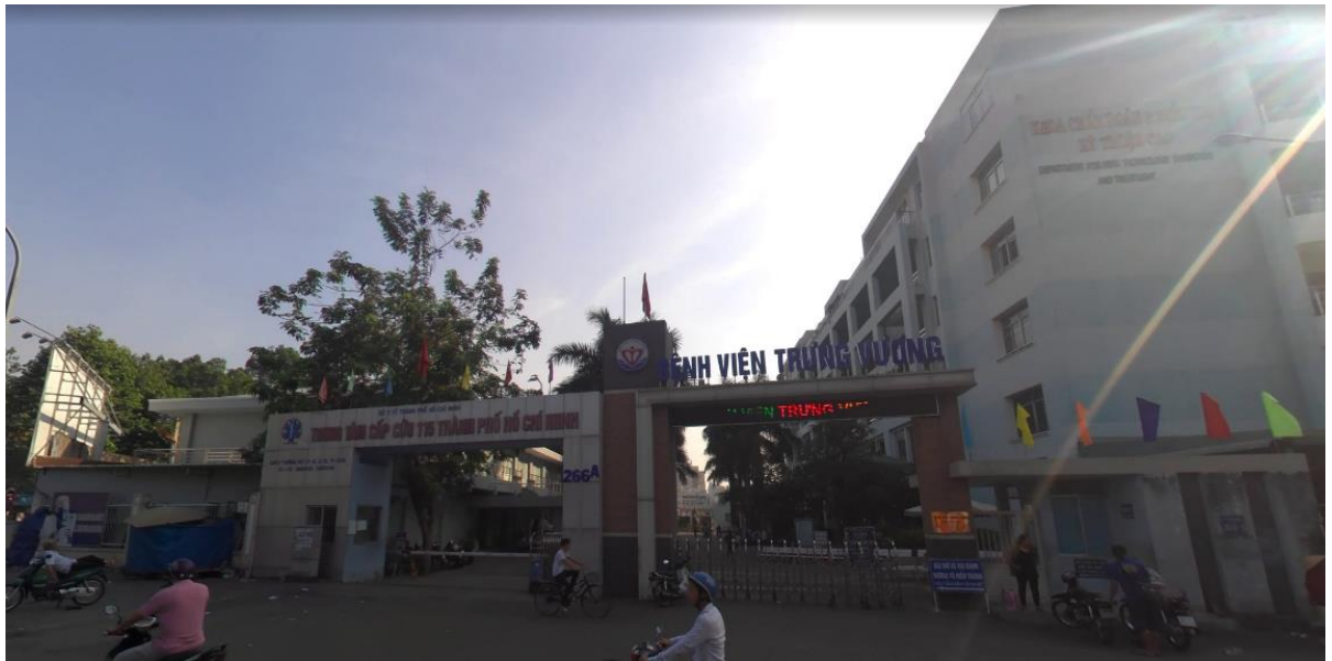
Figure 15 - Hôpital Trung Vuong Ho Chi Minh Ville - Google maps
