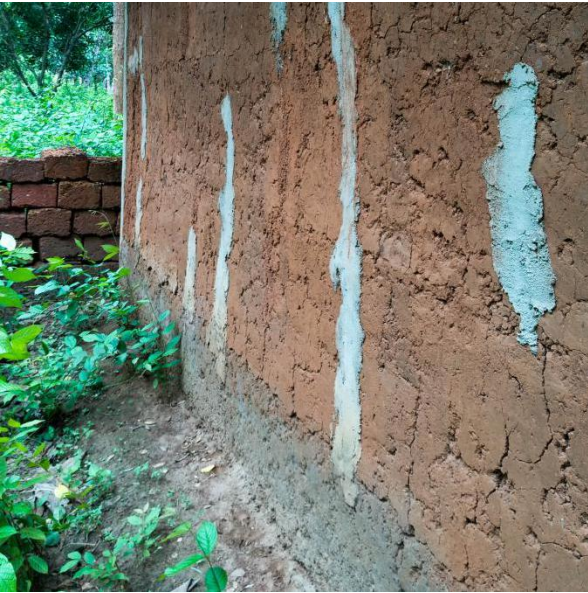
Observations: Base-course is greyish along the one facade. Repairs: Cracks and other repairs done in cement.
