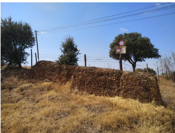
Image 150 and Image 151: Rammed-earth compound wall. Beja, Alentejo, 2018.
