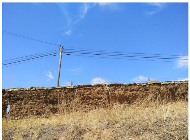
Image 150 and Image 151: Rammed-earth compound wall. Beja, Alentejo, 2018.
