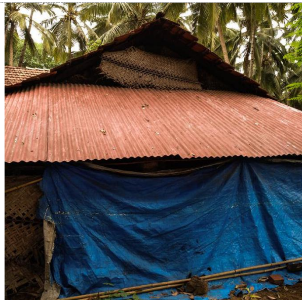
Maintenance and repairs: A woven coconut-frond ('molla') protects the gable from the sprays of rainwater.
