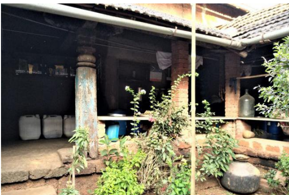
Distinct architectural details: Intricate wooden pillars once supported the veranda around the inner courtyard. Most of them are now replaced with fired-brick pillars.
