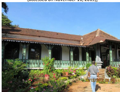
Image 60: The ‘ balkâmv ’ or ‘ balcão ’ of the Indo-Portuguese house. Margao, Salcete, South Goa, 2012.
