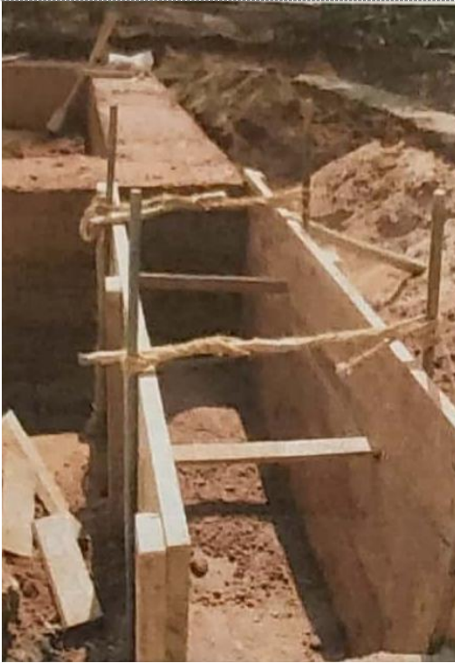
Banche traditionnelle et entretoise ('kani' in Konkani) [Source: Lobo, Earth in Architecture , 2006, p.42]
