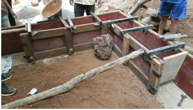
Recent rammed-earth form-works used in Goa.
