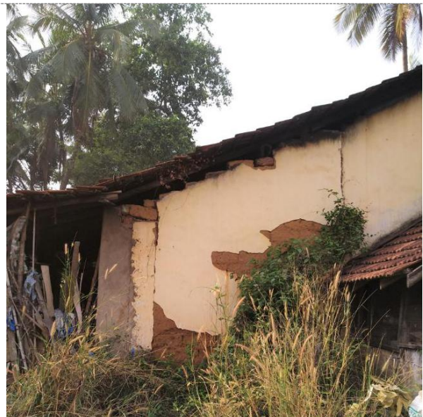
Damages incurred / problems faced: Flaking and falling plasters.
