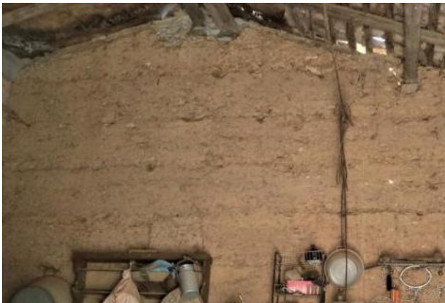
Image 170: Simple typology i.e. walls without mortar or other materials (Survey no. 1[1]).
