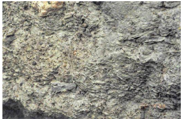
Distinct characteristics: Schist between rammed-earth 'lifts' on exterior walls.
