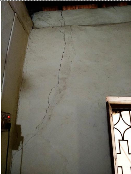
Damages incurred / problems faced: Cracks on the bedroom wall because of the weight of the roof.
