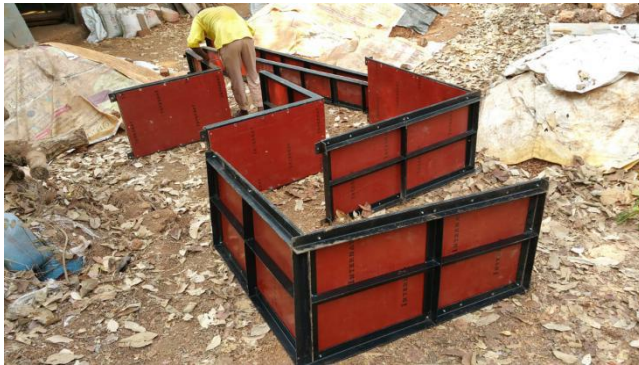
Recent rammed-earth form-works in Goa.
