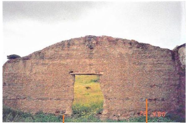
Schist and granite masonry.
