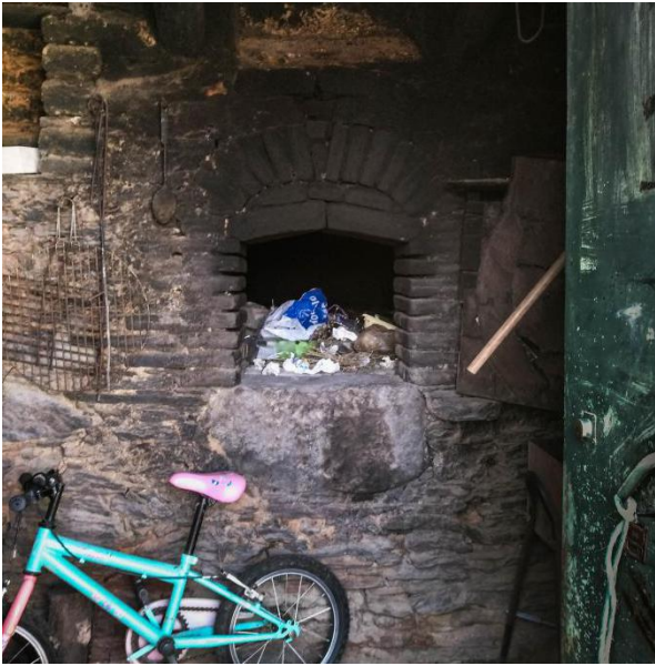
Oven inside the house.
