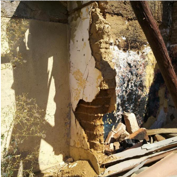
Distinct characteristics: There is an dividing wall, probably in adobe-bricks in the original building.
