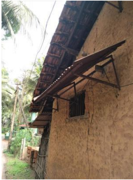
Image 120: Metal-sheet overhangs (Survey no. 9).
