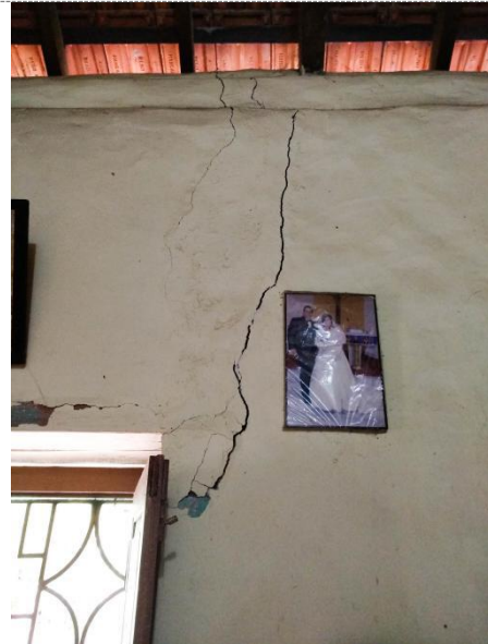
Damages incurred / problems faced: Cracks on the bedroom wall because of the weight of the roof.
