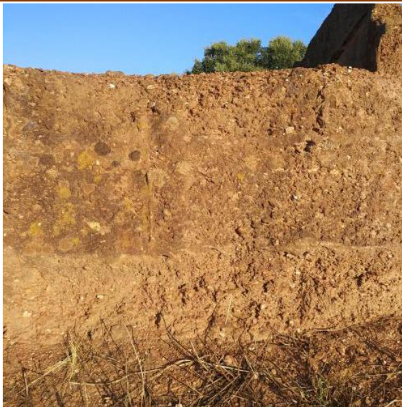
Image 180: Rammed-earth 'lifts' separated by earth and lime mortar (Survey no. 11[25]).
