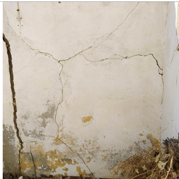
Damages incurred / problems faced: Cracks appeared and the walls began falling apart.
