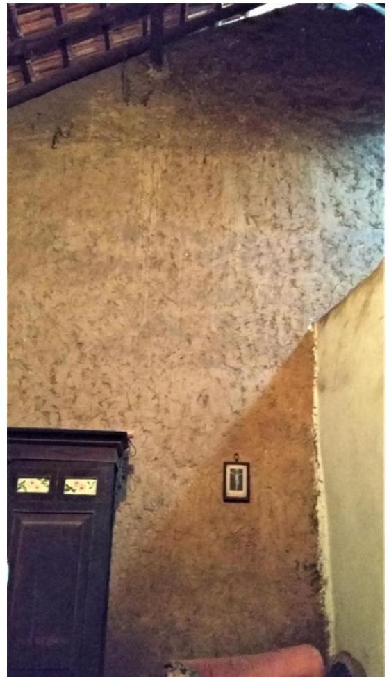
Image 67: 'Lift' joints visible (Survey no. 6).
