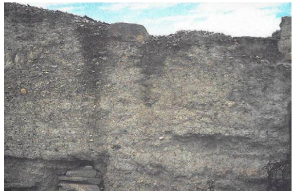
Use of stone in rammed-earth construction.
