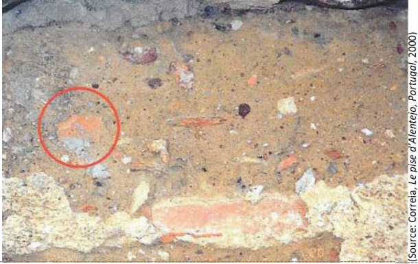
Earth used & Typology (original building)
