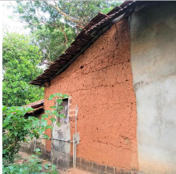
Distinct characteristics: Two, finer 'lifts' constitute the gable (other surveyed structures displayed a single 'lift' in the gable or 'lifts' with more height. Refer images in Survey nos. 1, 2, 6, 7).
