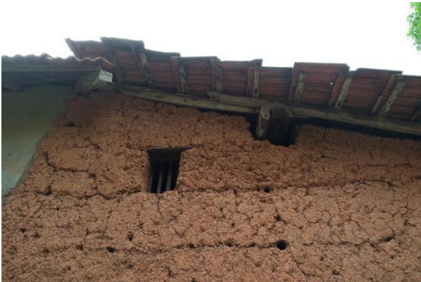
Distinct characteristics: Some holes on walls are well defined (suggesting cob construction with shutters?).
