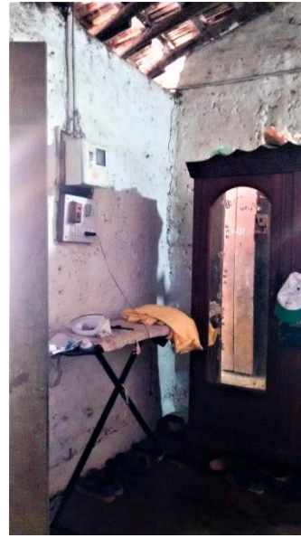
Plasters: Thin coat of lime on earthen walls (interior).
