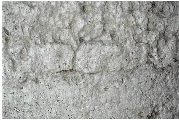
Distinct characteristics: There is a layer of adobe-bricks between the rammed-earth 'lifts'.
