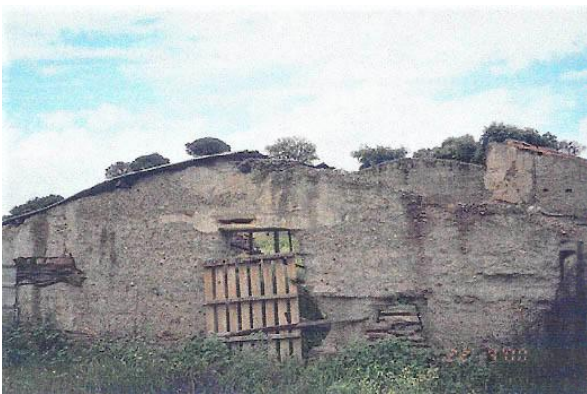
Use of stone in rammed-earth construction.
