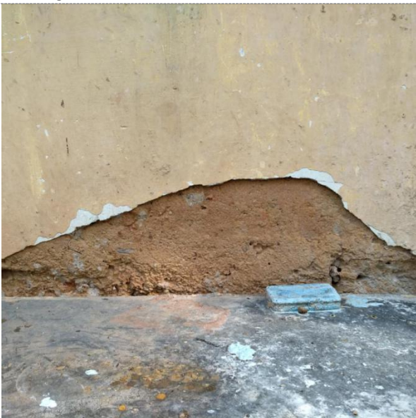
Damages incurred / problems faced: Flaking and falling plasters.
