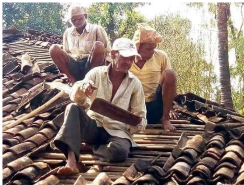
Image 116: Bamboo batons were used in case of 'Country-tile' roofs.
