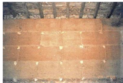
Holes left by the rammed-earth form-work covered with mortars.
