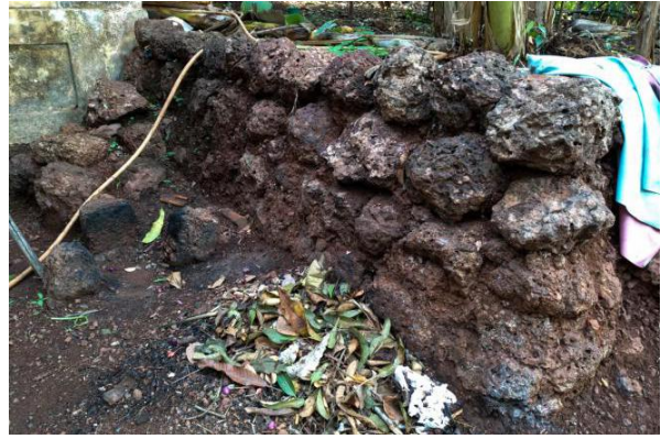
Distinct characteristics: Compound wall built with laterite-stones and earthen-mortars.
