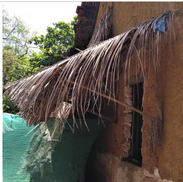
Maintenance and repairs: Every year before the monsoons, old palm-leaf overhangs are replaced with new ones.
