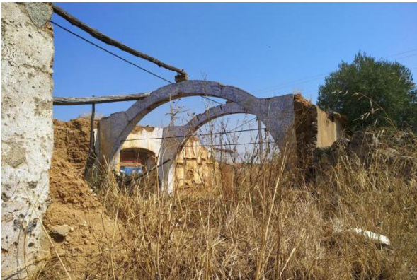
Distinct architectural details: Arches on the interior. Maintenance and repairs: Ties between arches.
