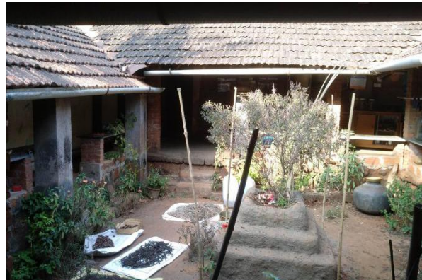
Openings: Inner courtyard.
