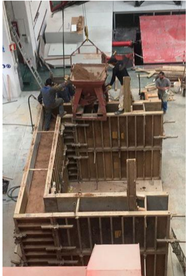
Modern rammed-earth form-work in Portugal.
