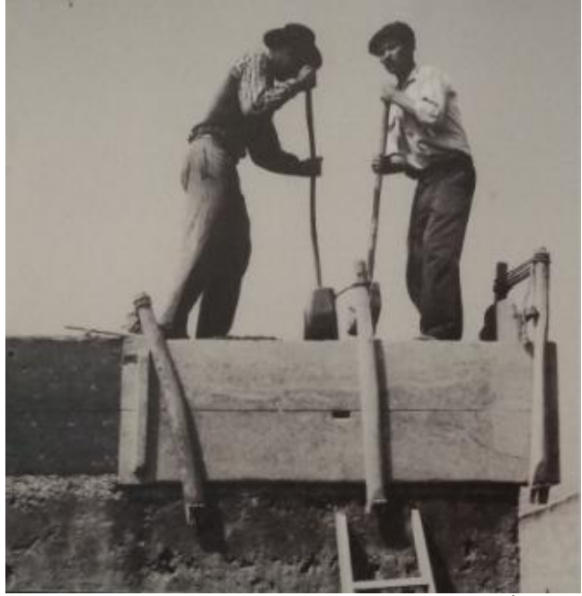
Traditional rammed-earth form-work used Aldeia da Luz in Évora before the 1950's. [Source: Panel at Museu da Luz, Luz, Évora, 2018]
