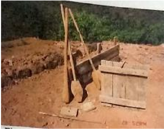
Form-work with bolts and spacers, and tools [Source: Lobo, Earth in Architecture , p.44]
