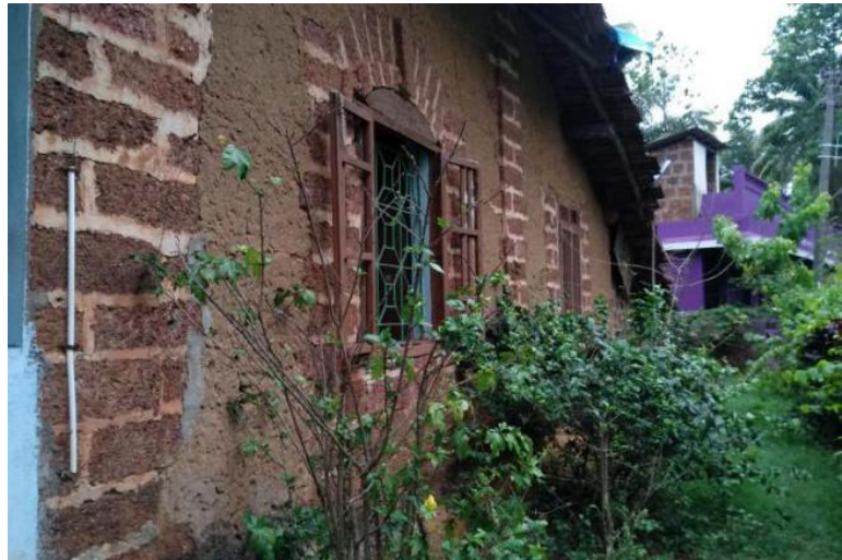
Image 71: Corners; a laterite-stone sits above the earthen base-course (Survey no. 1).
