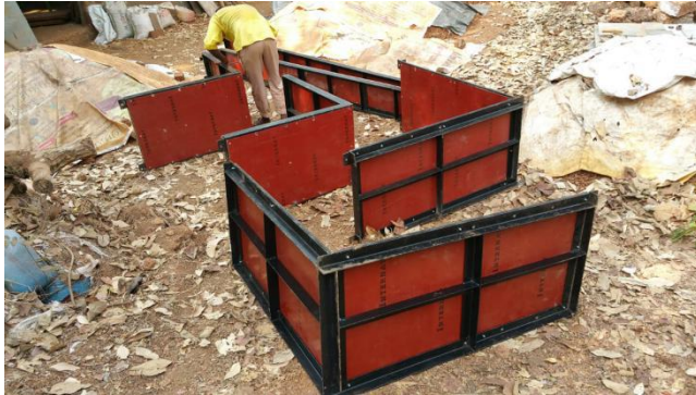
Recent rammed-earth form-works in Goa.
