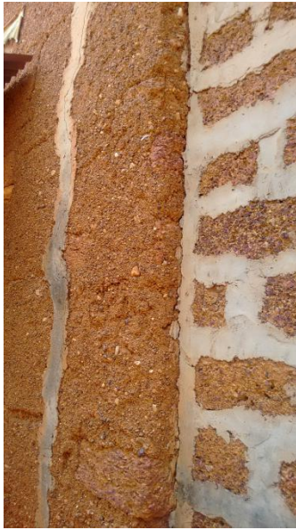
Corners: Mainly in earth, there are some laterite-stones.
