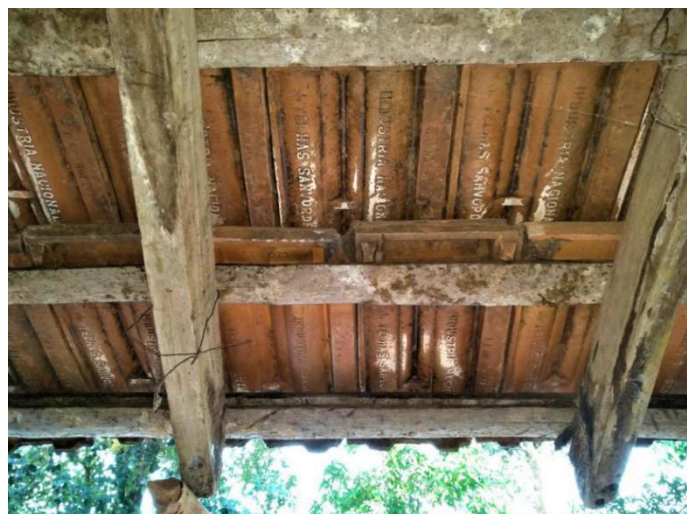
Image 127: Two, instead of one baton was fixed along the ends of the roof's framework (Survey no. 13).
