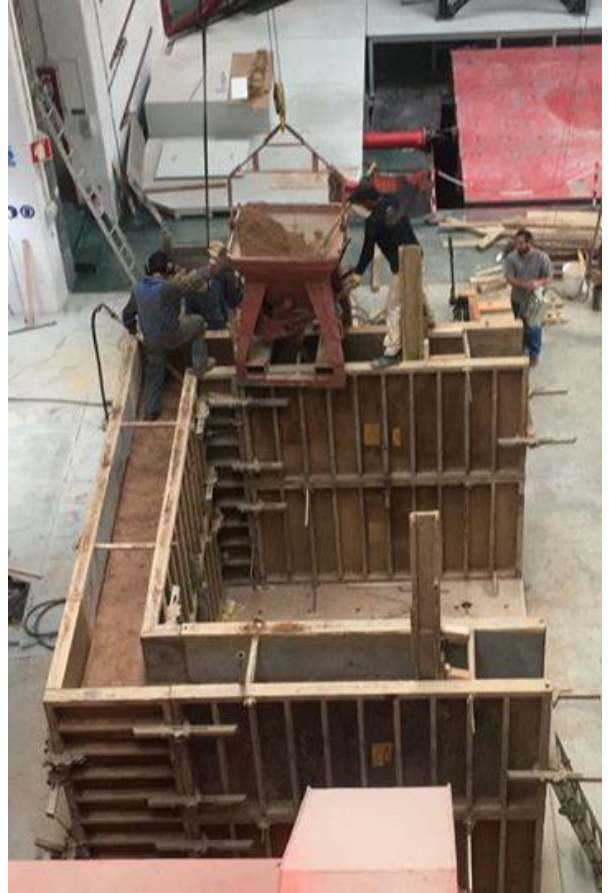
Modern rammed-earth form-work in Portugal.
