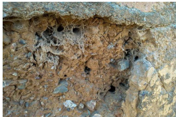
Damages incurred / problems faced: Mason-bee holes.
