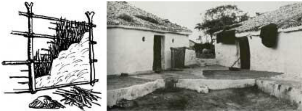
Image 29: Mud-and-wood or Wattle-and-daub constructions in Goa.
