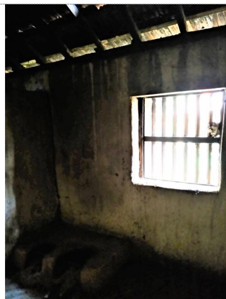
Maintenance and repairs: Cooking indoors on traditional wood-burning stoves gives out smoke; the heat and dryness makes the wood in the roof stronger, and keeps termites at bay.
