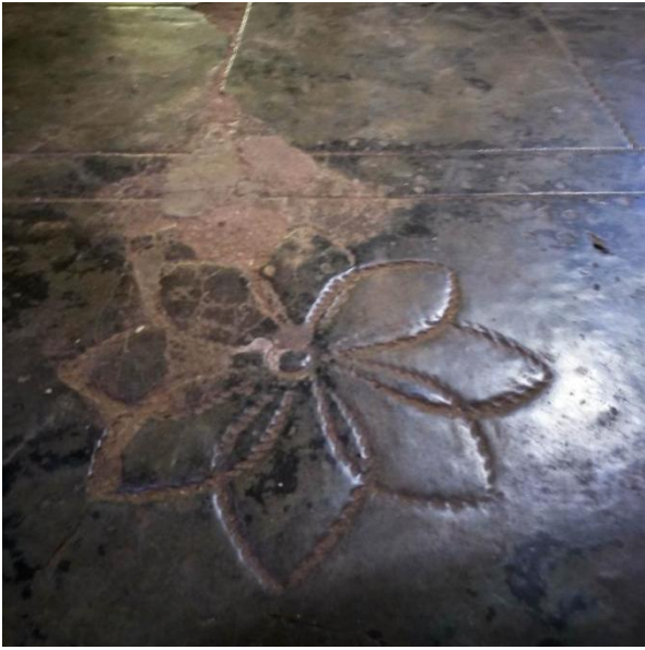
Flooring: Cement in hall; there are designs on the hall floor.
