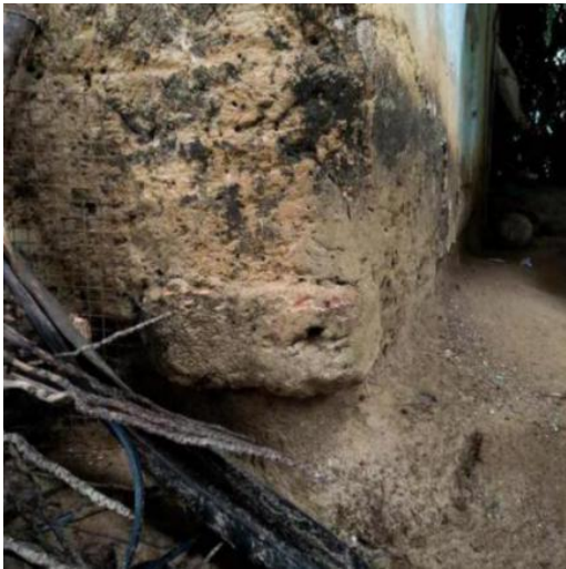
Image 71: Corners; a laterite-stone sits above the earthen base-course (Survey no. 1).
