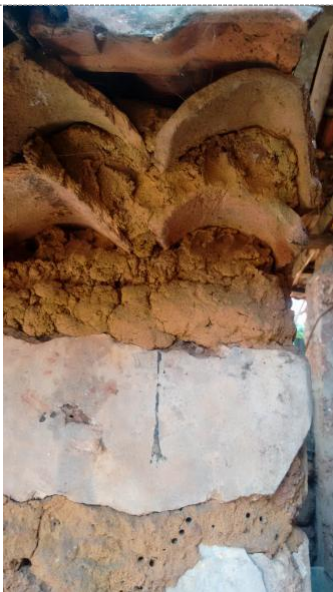
Maintenance and repairs: 'Menki-matti' (type of mud) used to touch-up the wall.
