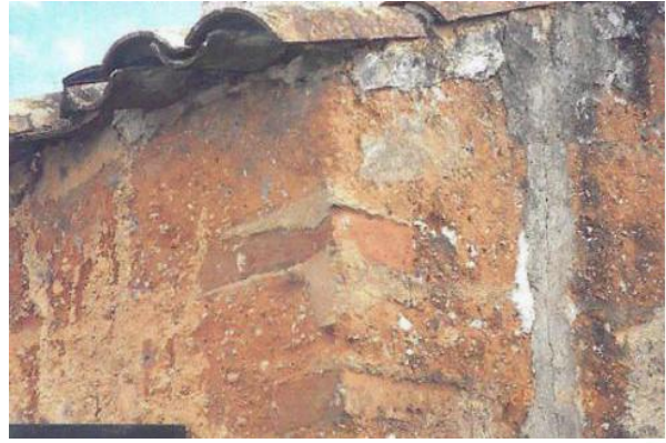
Corners: In rammed-earth and brick.
