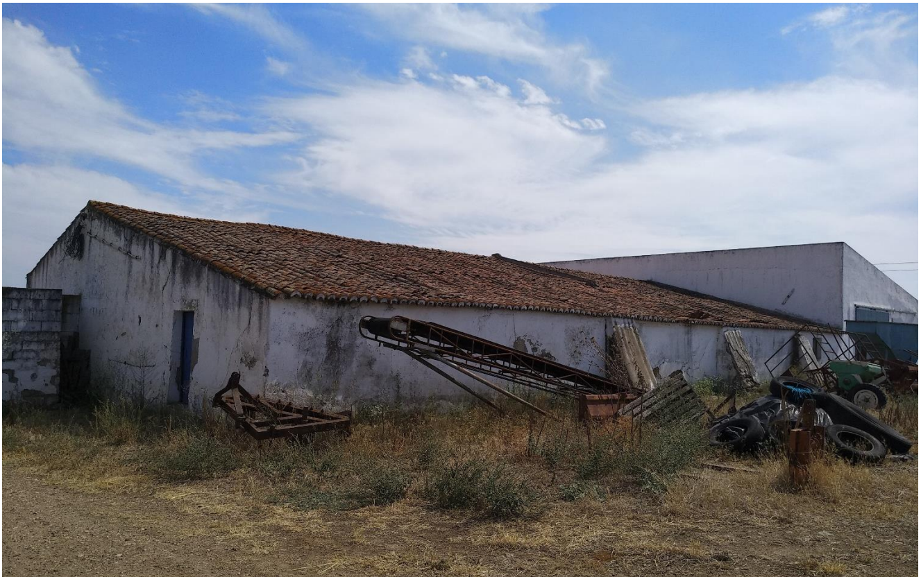
Figure 5: A 'Taipa' house with buttresses, which were probably built to keep the 'Taipa' wall from falling. Casa dos Trabalhadores do Monte Valvinagrinho, Moura
