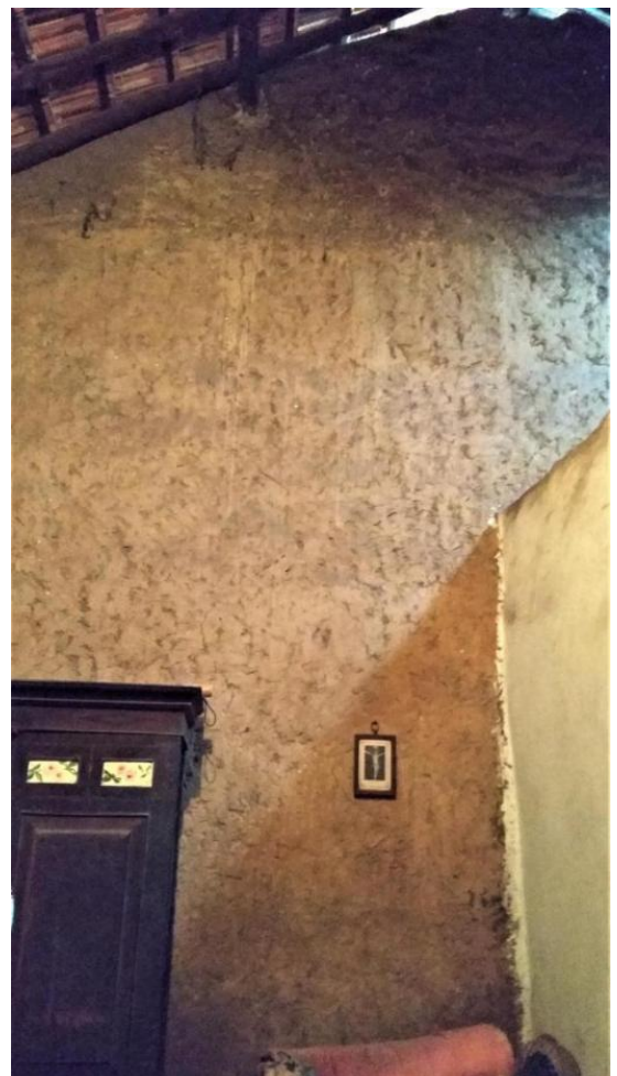
Image 67: 'Lift' joints visible (Survey no. 6).
