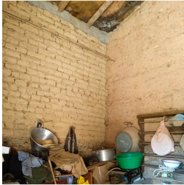
Distinct characteristics: Interior walls are in adobe-bricks.
