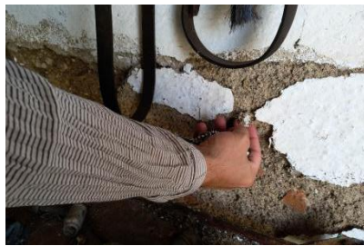
Damages incurred / problems faced: Warping, cracking and fallen plaster.
