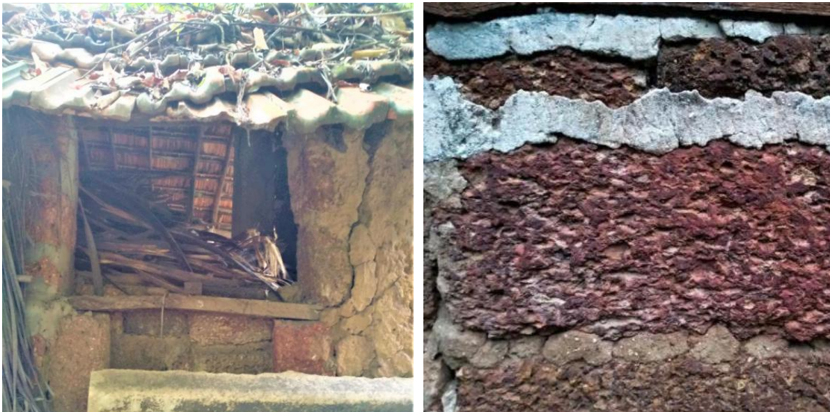
Image 134: Mortars were present in those parts of the walls that had laterite-stone masonry i.e. in the base-courses, window frames, corners, etc. (Survey no. 5).
