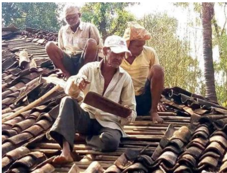
Image 116: Bamboo batons were used in case of 'Country-tile' roofs.
