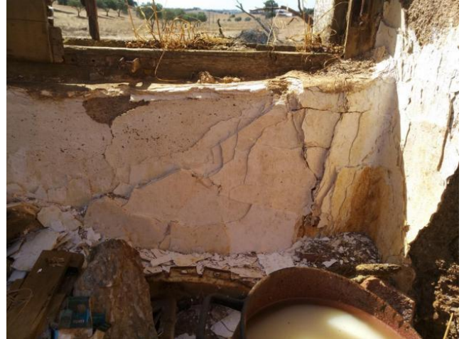
Traditionally, walls were whitewashed every 1-2 years. This created many paint layers, and thickened the walls over the years. Image 193: Wall in Moura, Beja, 2018. Image 194: A ruin of a house in Serpa, Beja, 2018.
