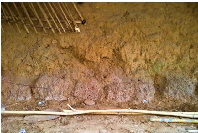
Damages incurred / problems faced: Erosion of the walls has created depressions above base-courses of external walls.
