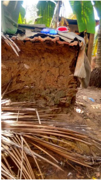
Front view of the wall.
