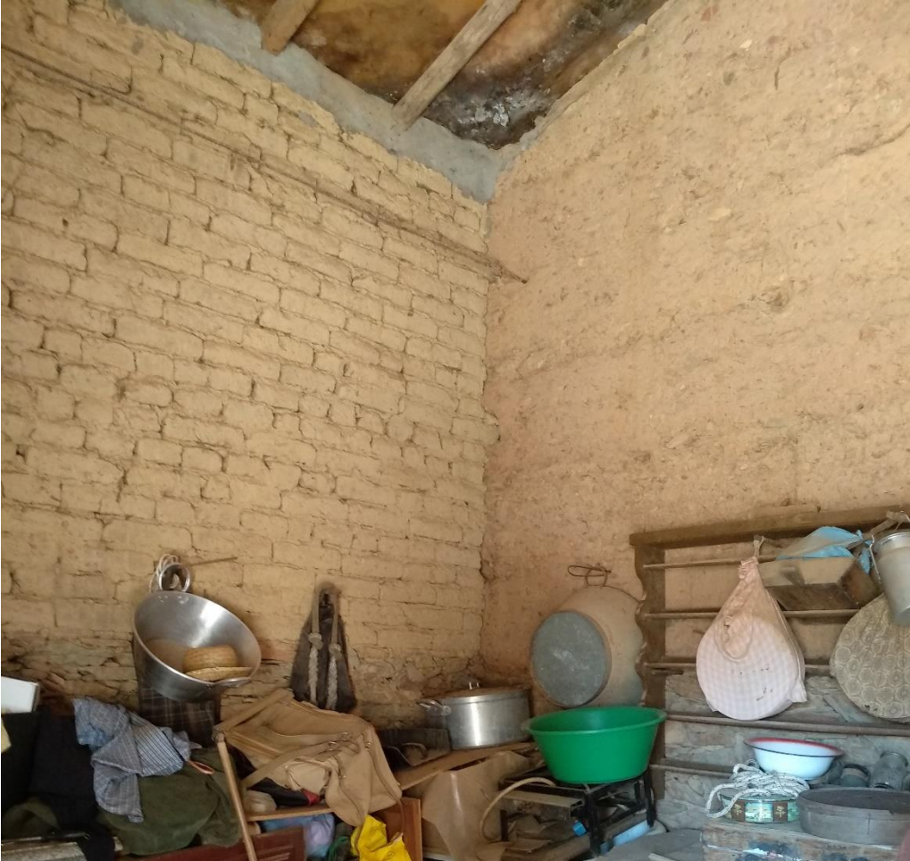
Figure 3: External wall of 'Taipa' and internal division wall in 'adobe' bricks.
