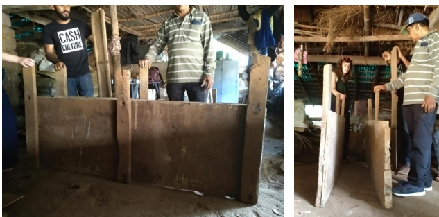
Parts of a recent rammed-earth form-work used in Goa (4 images). [Drawing by Lionel Afonso]
