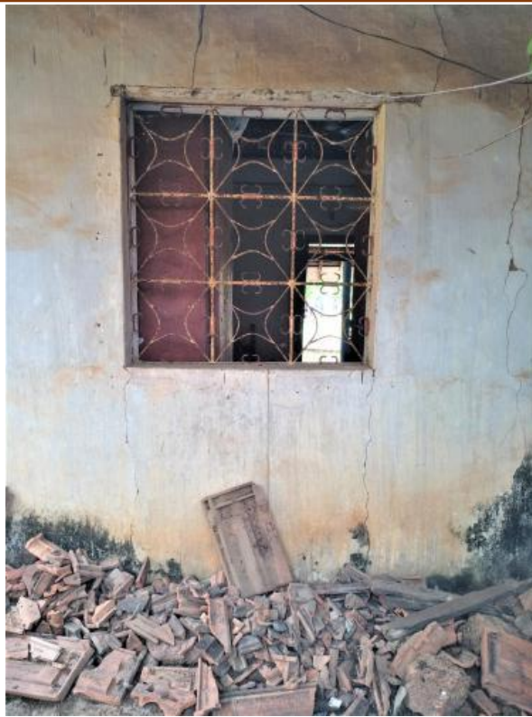
Image 138: The lack of support provided by rotting lintels caused the roof to put pressure on the wall, and created many cracks around the window (Survey no. 7).
