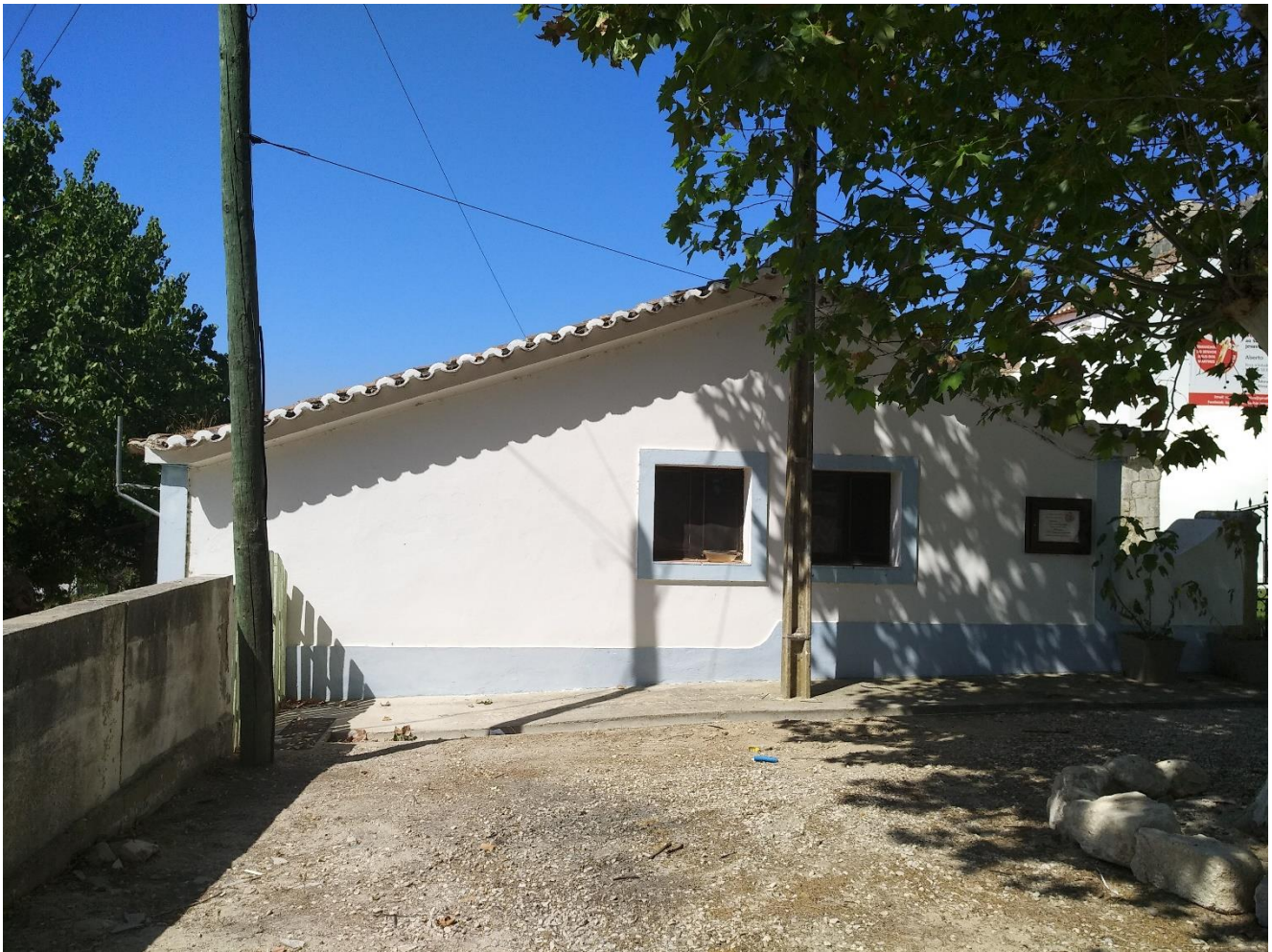
Figure 8: A recently plastered 'Taipa' house Casas dos Romeiros, Alcácer do Sal
