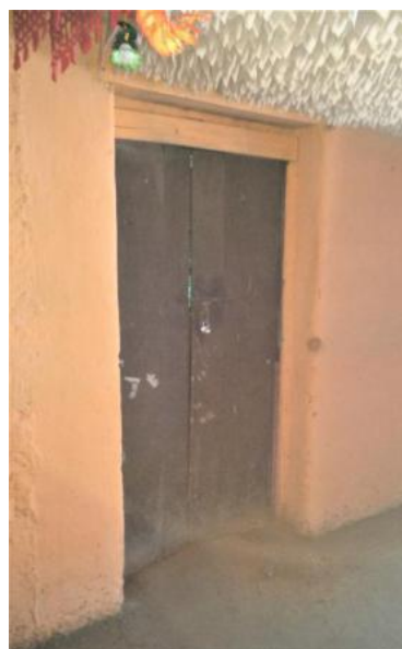
Image 92: Lintels of doors and windows were mostly slanted, and opened up to the interior of the house (Survey no. 3a). Image 93: In a few cases, the lintels were simply placed horizontally (Survey no. 12).
