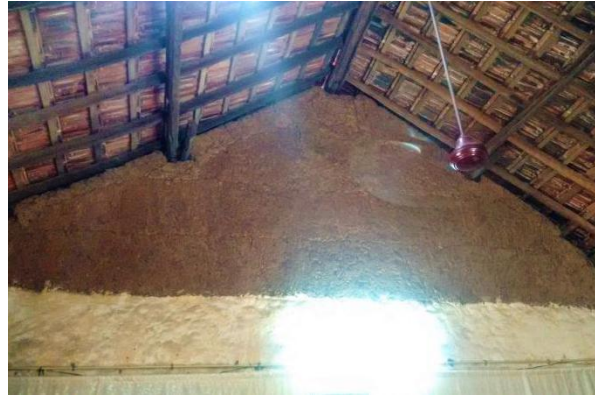
Observations: An additional layer of earth caps the roof-line. Looks like this was done after the roof was installed in order to secure the rafters to the wall. (Also refer image in 'Typology' section.)
