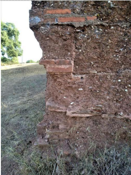
Base-course: 0.30m; in stone. Corners: In rammed-earth and fired-bricks. Distinct characteristics: Evidence of schist between the rammed-earth 'lifts'.
