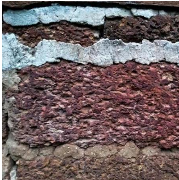
Image 134: Mortars were present in those parts of the walls that had laterite-stone masonry i.e. in the base-courses, window frames, corners, etc. (Survey no. 5).
