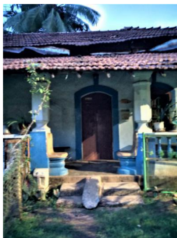
Image 86: Almost all the structures visited for this study had verandas, porches and/or 'sopos'. Some verandas had inbuilt masonry seats. (Survey no. 3a).
