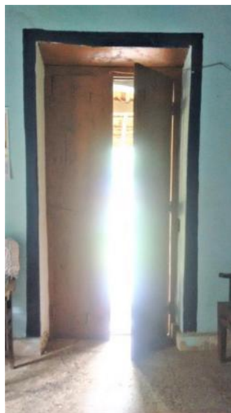
Image 92: Lintels of doors and windows were mostly slanted, and opened up to the interior of the house (Survey no. 3a). Image 93: In a few cases, the lintels were simply placed horizontally (Survey no. 12).
