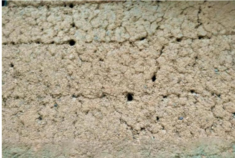
Image 70: Holes along the horizontal 'lift' joints, which perhaps indicates the use of form-work in cob construction (Survey no. 11).
