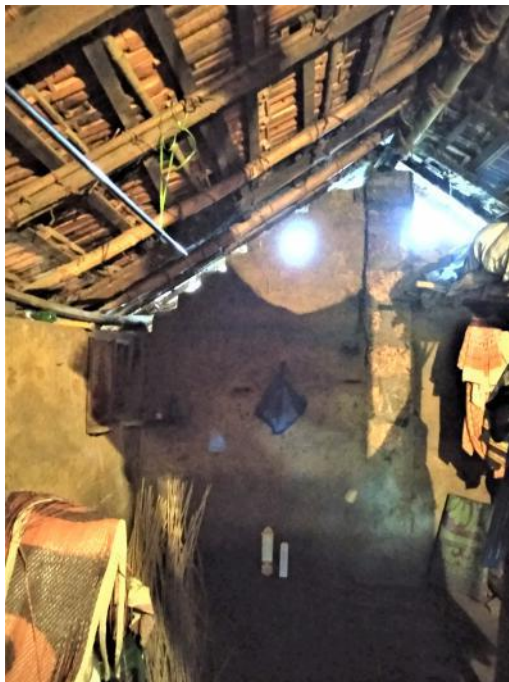
Image 117: Sometimes, bamboo and other similar materials were used even in the case of 'Mangalore-tiles' roof framework as well (Survey no. 4).
