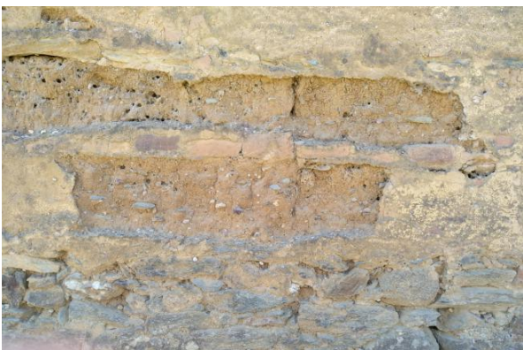
Damages incurred / problems faced: Mason-bee holes.
