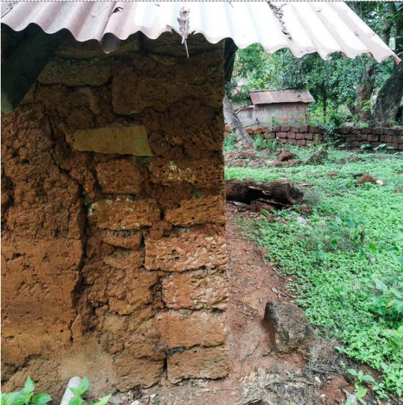
Observations: The laterite masonry in the corners has earthen or cement mortars. It is hard to say whether these corners are part of the original construction or a later addition.
