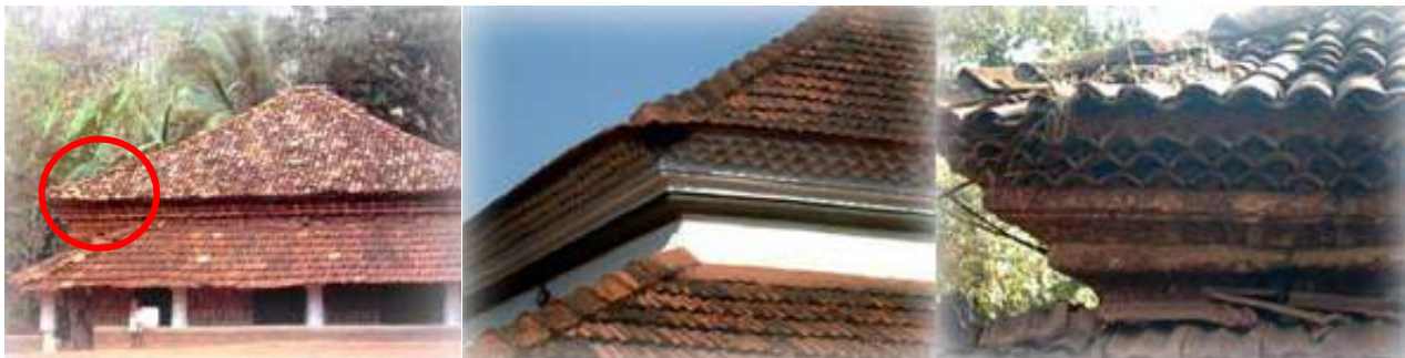
Image 55, Image 56 and Image 57: Corbelling made with 'Country-tiles'.
