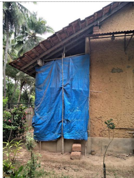
Observations: Metal overhangs and tarpaulins protect walls from rainwater.
