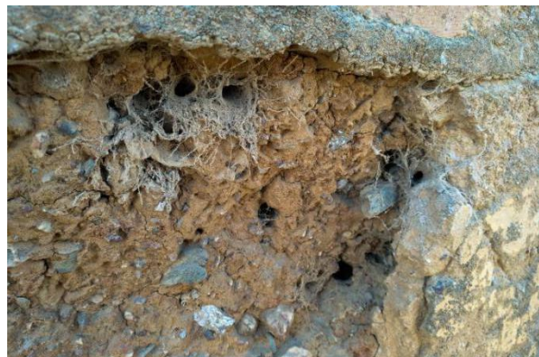
Damages incurred / problems faced: Mason-bee holes.
