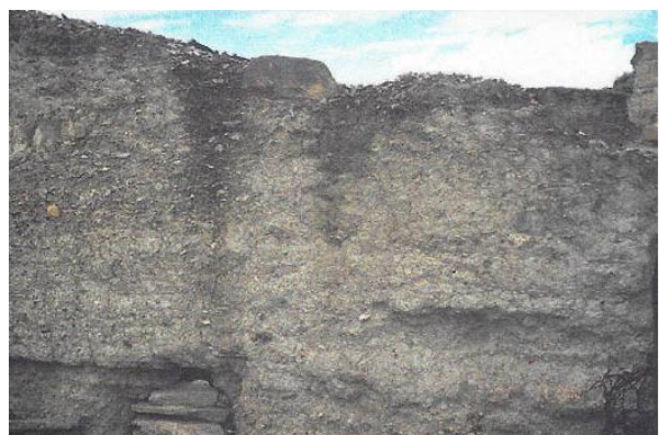
Use of stone in rammed-earth construction.
