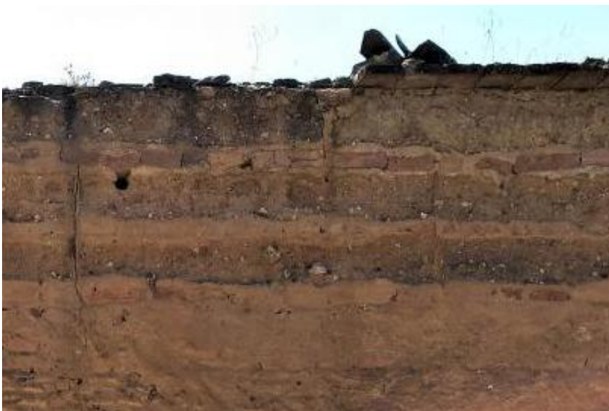
Image 172: Two rammed-earth layers within each block, separated by a layer of mortar + fired-brick + mortar (Survey no. 3[9]).
