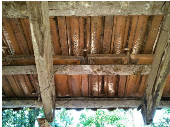
Image 127: Two, instead of one baton was fixed along the ends of the roof's framework (Survey no. 13). Image 128: Splits of the beetle-nut tree were used as batons. Two batons were used along the roof-line. (Survey no. 12).
