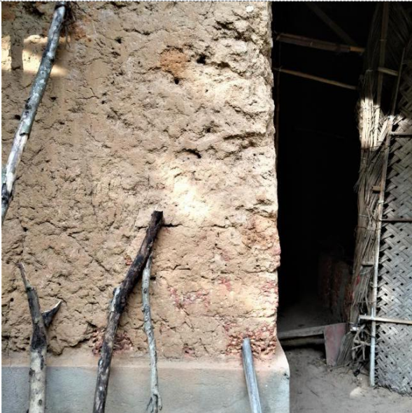
Corners: In laterite masonry on lower walls; earth on higher parts of the walls.
