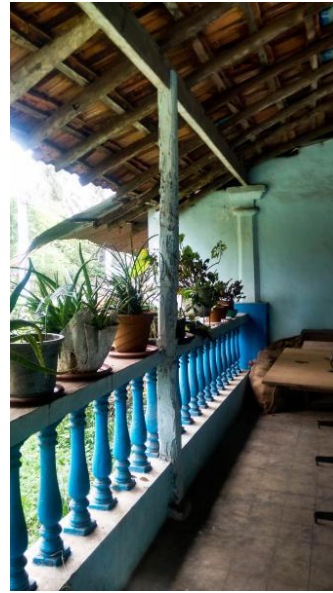
Distinct architectural details: Wooden pillar in the veranda.
