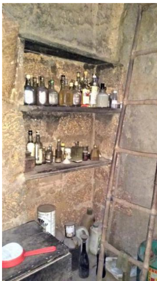
Image 101: Provisions for niches and shelves in walls were made at the time of construction (Survey no. 15).
