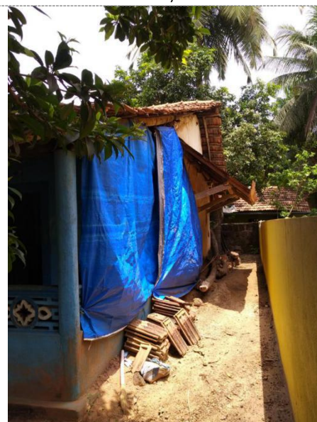
Maintenance and repairs: Tarpaulins covers are usually mounted before the monsoons and removed after the monsoons.
