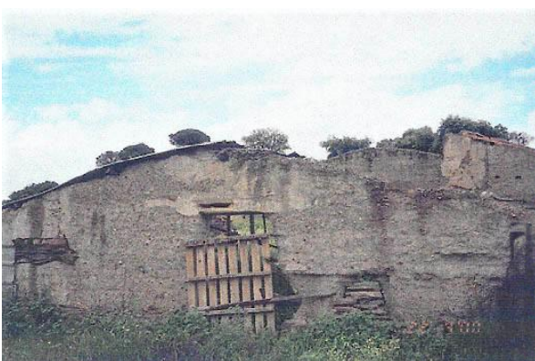
Use of stone in rammed-earth construction.
