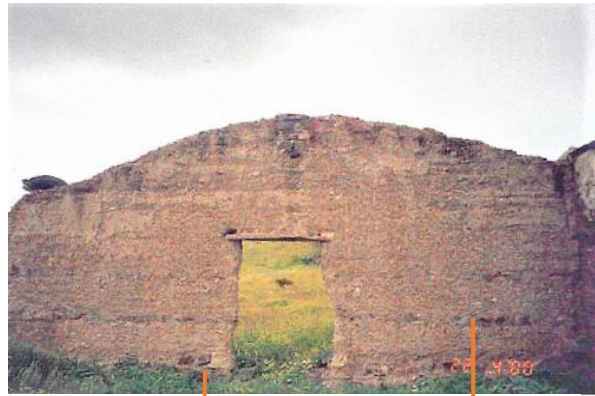
Schist and granite masonry.
