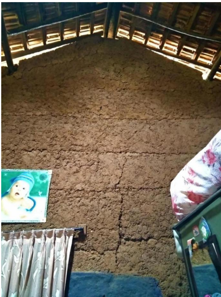
Image 67: 'Lift' joints visible (Survey no. 6).
