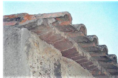
Overhangs, houses in Portugal.
