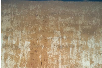
Holes left by the rammed-earth form-work covered with earth.
