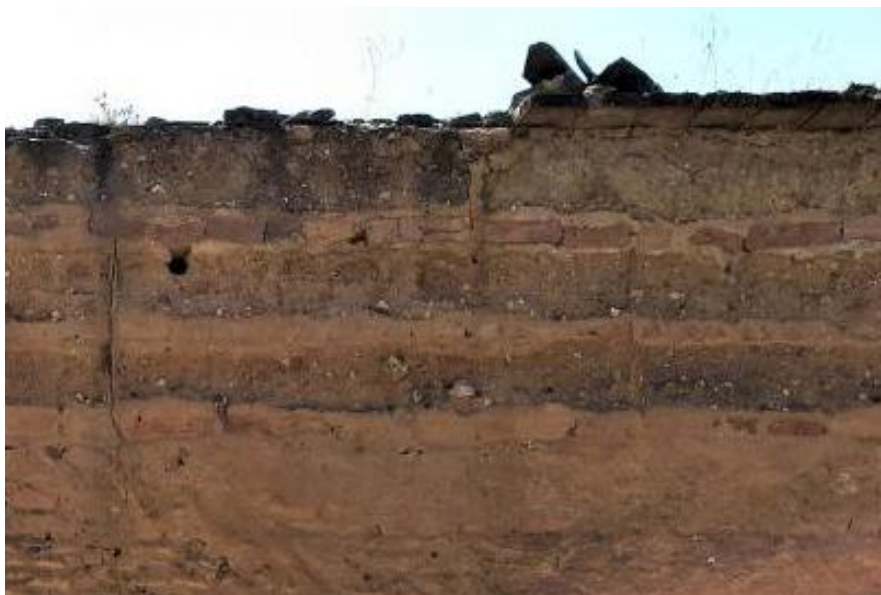
Image 172: Two rammed-earth layers within each block, separated by a layer of mortar + fired-brick + mortar (Survey no. 3[9]).
