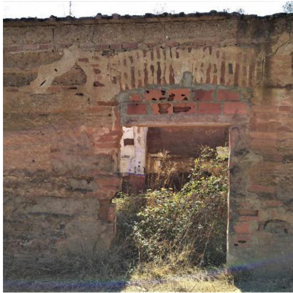
Base-course: In schist and granite masonry. Use of fired-bricks along door frame.
