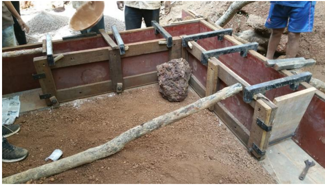
Recent rammed-earth form-works used in Goa.
