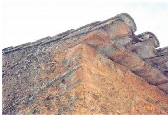
Image 189: Fired-brick overhangs.
