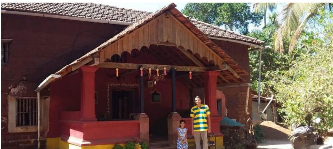
Image 131: Eaves (Survey no. 15). [Source: https://www.tanshikarspicefarm.com/# ]
