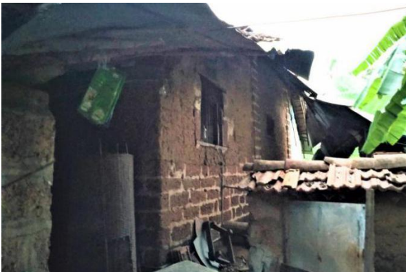
Distinct architectural details: Kitchen wall is partly built in laterite-masonry, whereas the hall is not. (Back in time, service rooms such as kitchens and storerooms were built with less expensive materials as compared to halls and bedrooms.)
