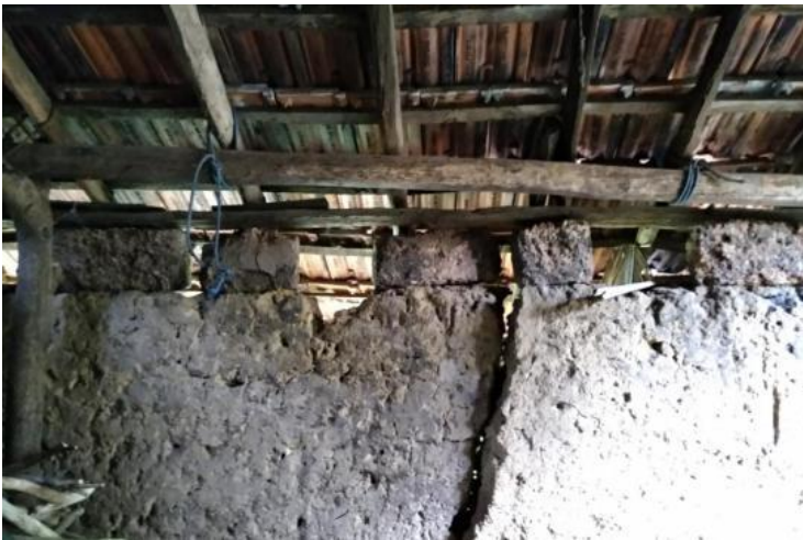
Image 112 and Image 113: On some wall tops, laterite-stones were placed at random intervals, on which a wooden plate or rafter was placed (Survey nos. 5, 8).
