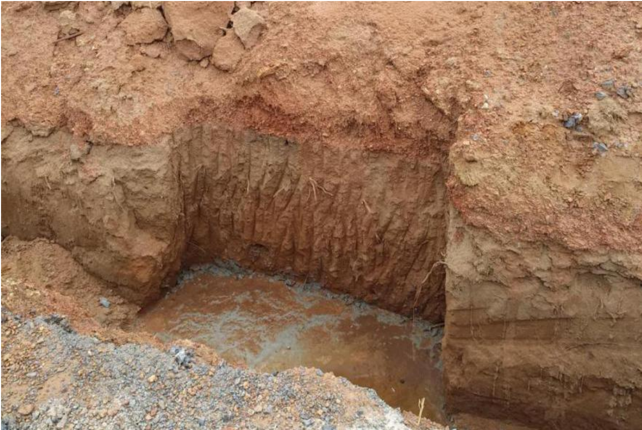
Image 69: Generally, top soil tends to be more sandy with more rubble.
