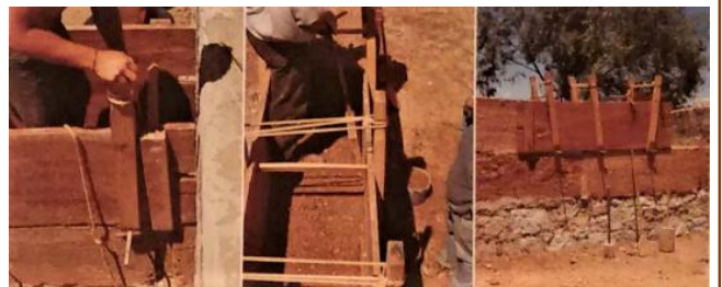
Traditional rammed-earth form-work of Alentejo
