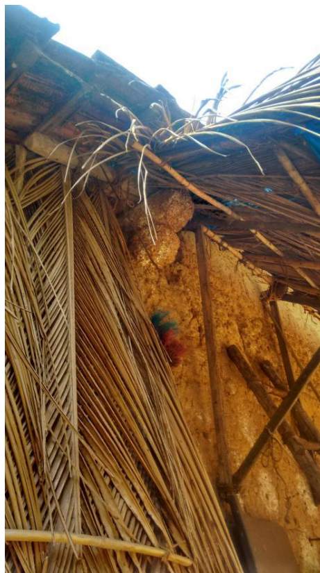
Image 123: Two decoratively cut laterite-stones that jutted-out from the wall top were probably meant to support the roof framework, but sometimes aided in holding the overhangs as well. (Survey no. 1).
