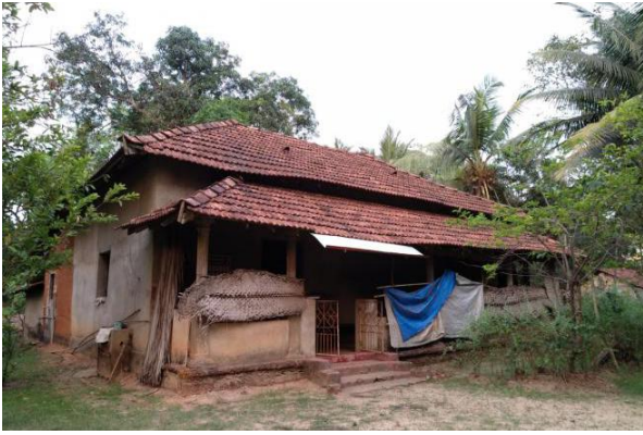
Distinct architectural details: Decorative laterite masonry base-course on front facade. Maintenance and repairs: Taraulins, coconut palms and woven coconut-palms protect the veranda from rainwater.
