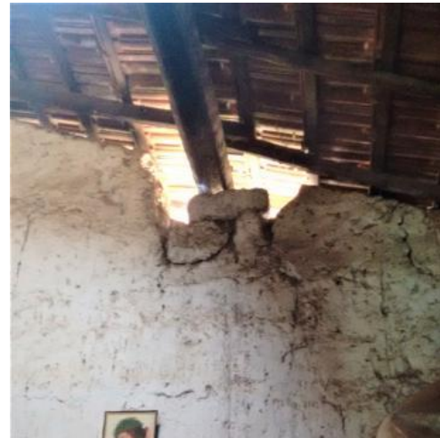
Image 112 and Image 113: On some wall tops, laterite-stones were placed at random intervals, on which a wooden plate or rafter was placed (Survey nos. 5, 8).
