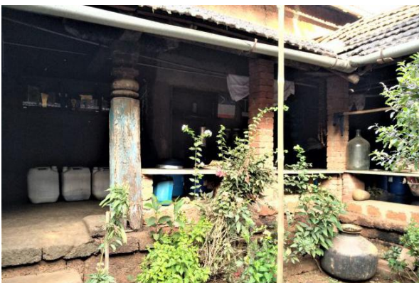
Distinct architectural details: Intricate wooden pillars once supported the veranda around the inner courtyard. Most of them are now replaced with fired-brick pillars.
