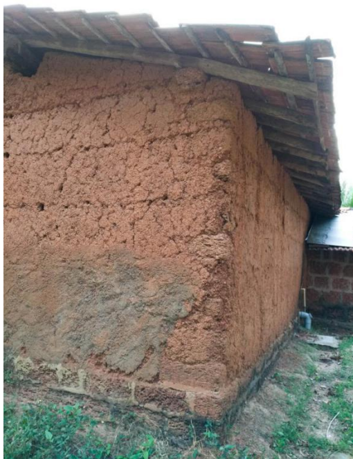
Image 73: Corners; earth with laterite-stones at intervals (Survey no. 11).
