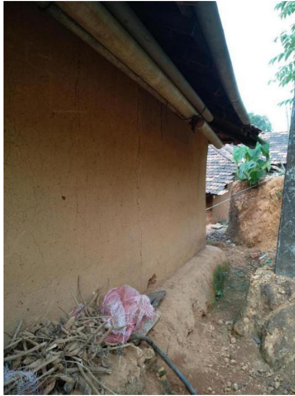
Image 75: Rammed-earth 'lifts' could not be determined as the walls displayed an uniform texture. The walls were beaten with a wooden baton during construction to compact them and realise a neat finish (Survey no. 13).
