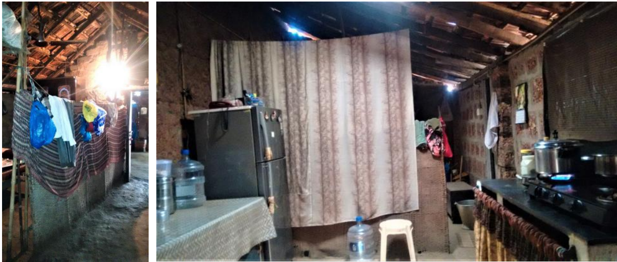
Image 104: Room dividers made with woven mats (Survey nos. 4, 6).
