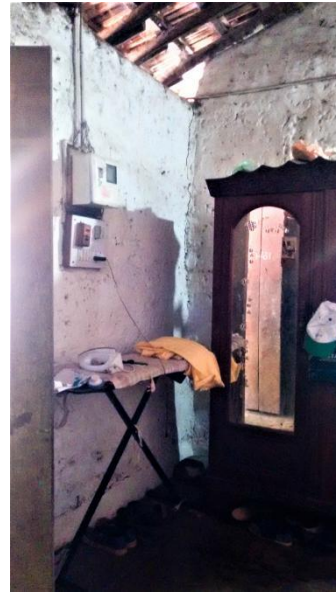
Plasters: Thin coat of lime on earthen walls (interior).
