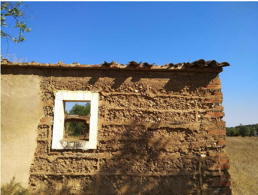
Figure 4: Typology of a 'Taipa' house in Serpa.
