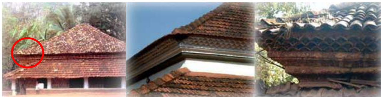
Image 55, Image 56 and Image 57: Corbelling made with 'Country-tiles'.
