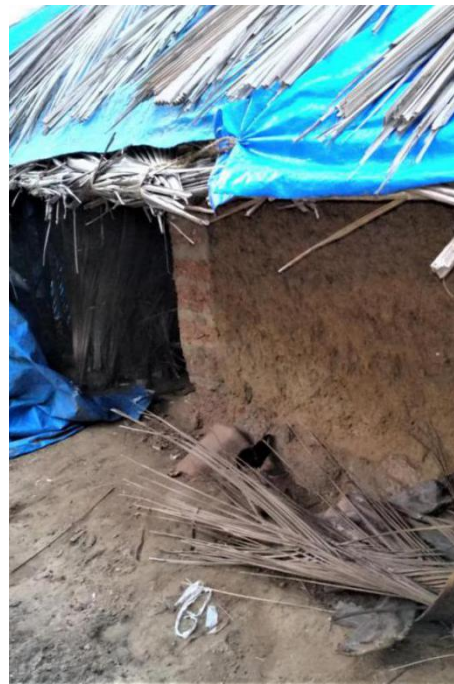
Image 73: Corners; earth with laterite-stones at intervals (Survey no. 11).
