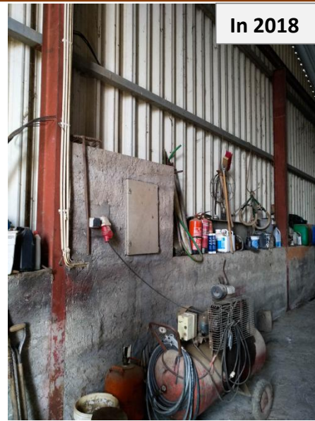
Interior view after the structure was rebuilt.
