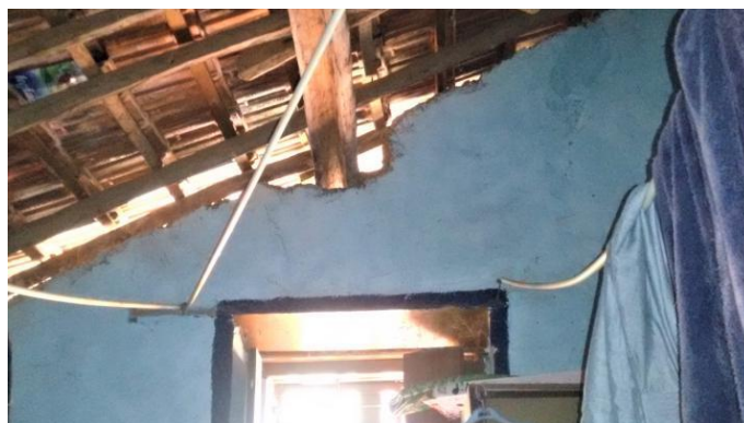
Image 114: Sometimes, the wooden plate directly rested on the top of the wall, and held the framework. On gable tops, crude holes were usually made to accommodate the rafters (Survey no. 3a).
