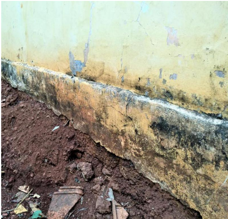
Image 79: Evidence of laterite masonry base-course (Survey no. 14).
