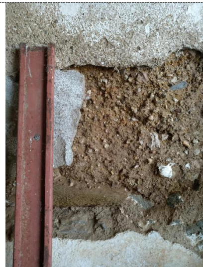
Damages incurred / problems faced: Warping, cracking and fallen plaster.
