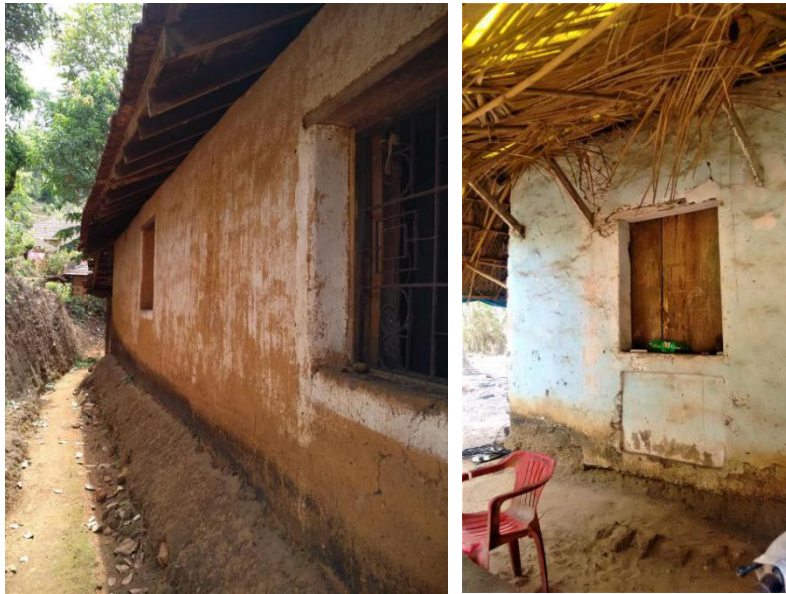
Image 87: A small, earthen gradient covered the foot of external walls (Survey no. 12).
