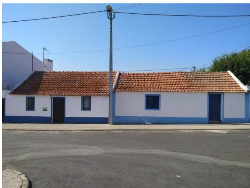
Image 153: Painting base-courses and the frames of openings in traditional colours continues even today. However, today synthetic paints ( ‘tinta’ ), rather than pigments are used. Alcácer do Sal, Setúbal, Alentejo, 2018.
