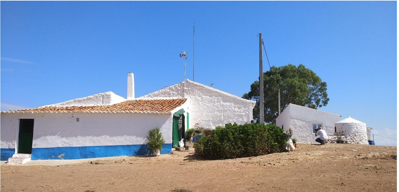
Figure 6: Whitewashed 'Taipa' walls of Pedreiro , António Martins Inácio's house. ' Pedreiro ' is the Portuguese word for 'mason'. António Martins Inácio is a traditional mud-mason. Serpa
