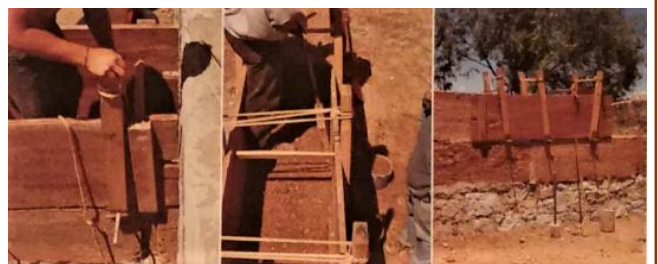
Traditional rammed-earth form-work of Alentejo
