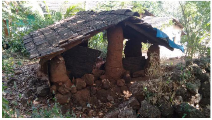
Outhouses, roof supported on earthen pillars.
