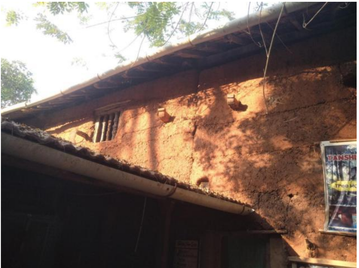
Image 121: Wooden pegs along the lengths of some façade walls (Survey no. 15).
