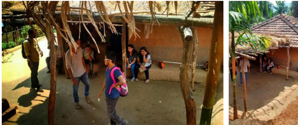
Image 58 and Image 59: The ‘ padvi ’ or ‘ pakadi ’ i.e. the lean-to with masonry seats, along the facades of rural Goan houses eventually evolved into a veranda with decorative railings and colonnades under the Portuguese influence, and took the form of a ‘ balkâmv ’ or ‘ balcão ’.
