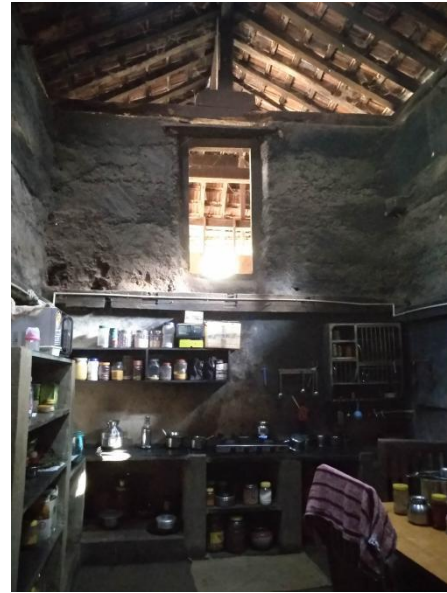
Restorations and/or interventions: Earlier, there used to be a loft in the kitchen, which is now taken-off. The door to the loft can still be seen.
