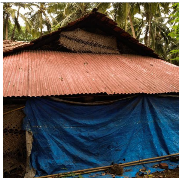
Maintenance and repairs: A woven coconut-frond ('molla') protects the gable from the sprays of rainwater.
