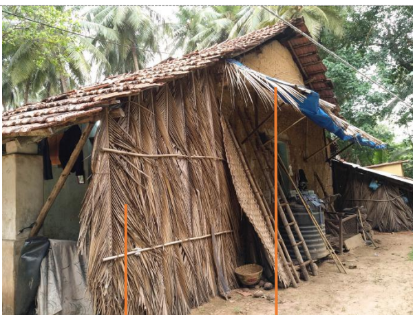
Palm-leaf barrier along walls ('dollo').
