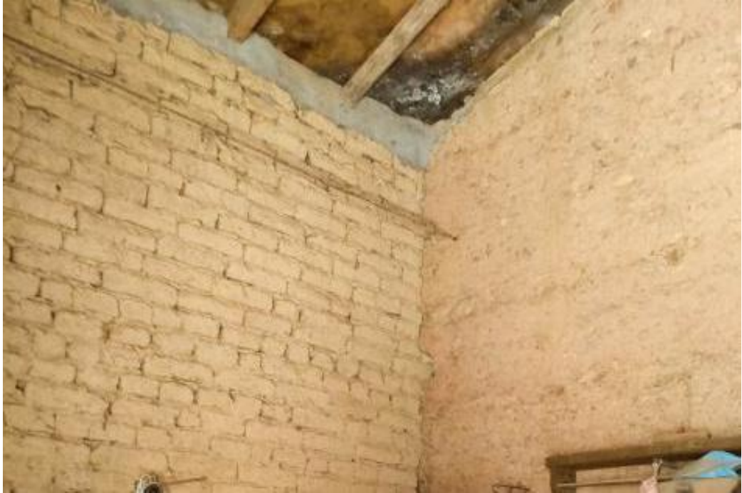
Image 187: External walls in rammed-earth and internal walls in adobe-bricks (Survey no. 1[1]).
