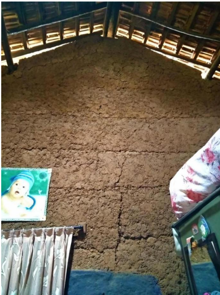
Image 67: 'Lift' joints visible (Survey no. 6).
