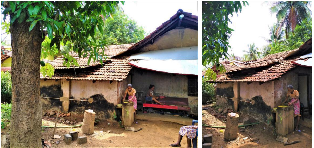
Image 107 and Image 108: A flap opened in the roof, creating an opening (Survey no. 7).
