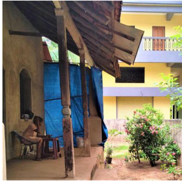
Distinct architectural details: Decorative wooden pillars support the roof in the veranda.
