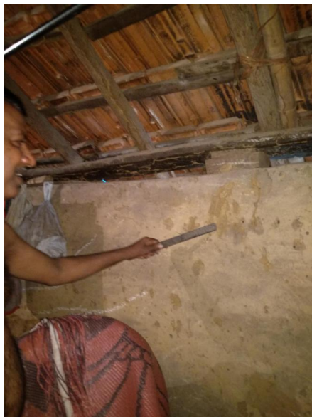
Image 140: An owner demonstrating how to manually break earthen-nests built by insects on interior walls (Survey no. 4).
