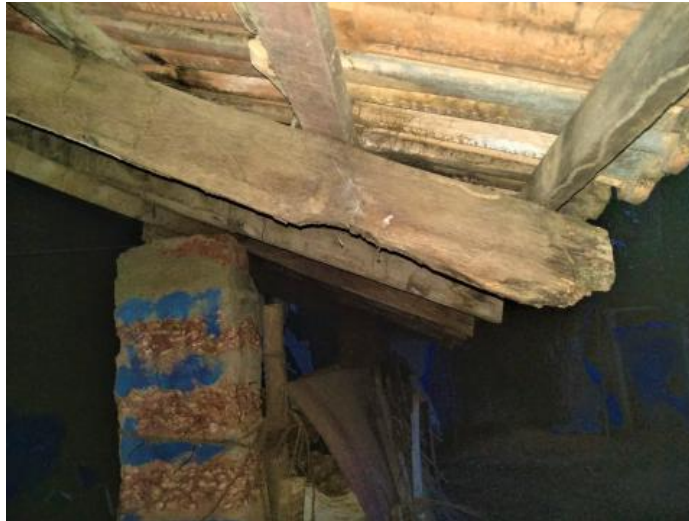
The last baton along the edge of the roof is placed with the smaller side resting on the rafters. Image 124 and Image 125: (Survey no. 8). Image 126: (Survey no. 3a).
