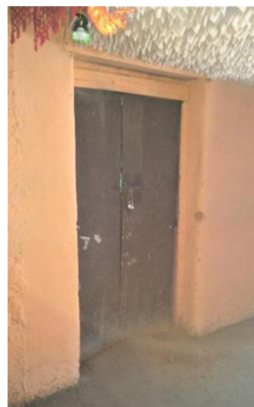
Image 92: Lintels of doors and windows were mostly slanted, and opened up to the interior of the house (Survey no. 3a). Image 93: In a few cases, the lintels were simply placed horizontally (Survey no. 12).
