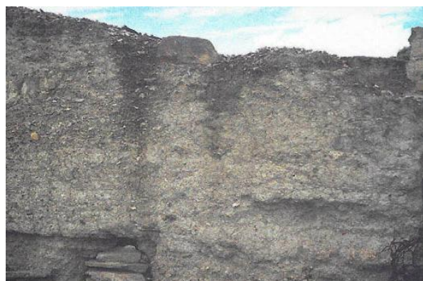
Use of stone in rammed-earth construction.
