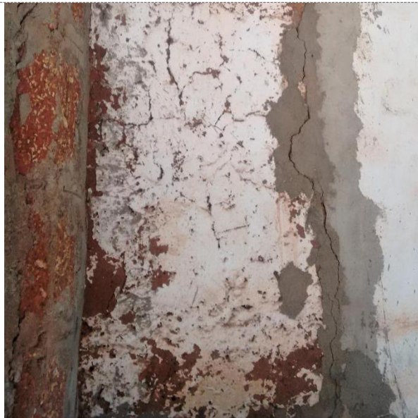
Plasters: A coat of lime or paint on south facade.
