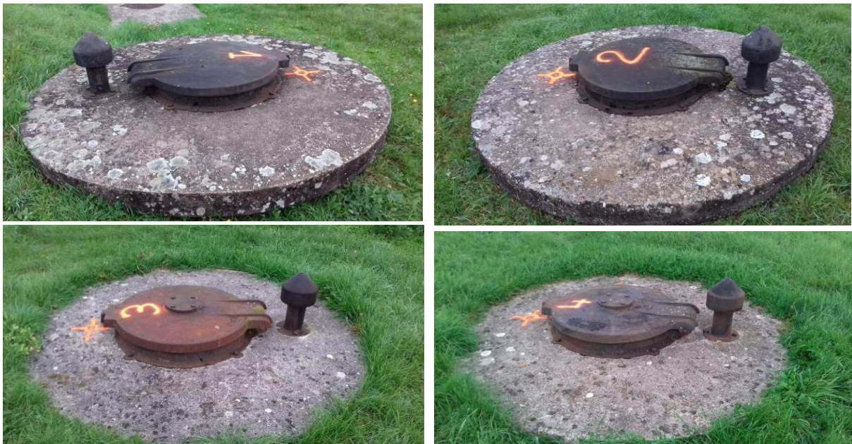
Figure 3 Captage Larente Logerot
