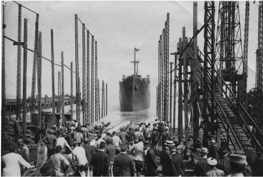
Chantiers Dubigeon XXe siècle
