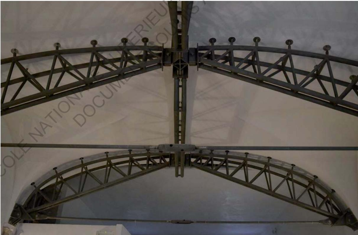
**FIGURE 59 : RESTAURATION D'UNE VOÛTE PAR AJOUT D'UNE STRUCTURE LA SUPPORTANT**
