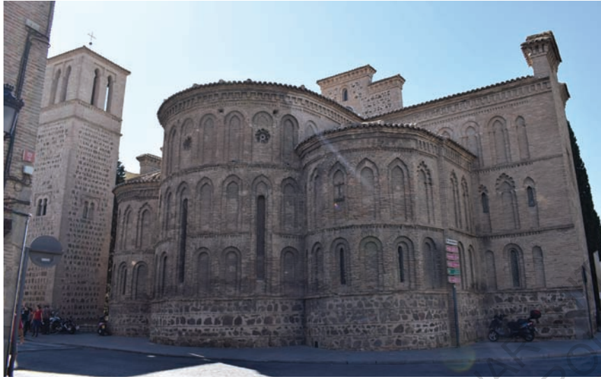
Figure 238: Eglise Santiago del Arrabal, Tolède, architecture mudéjare tolédane.
