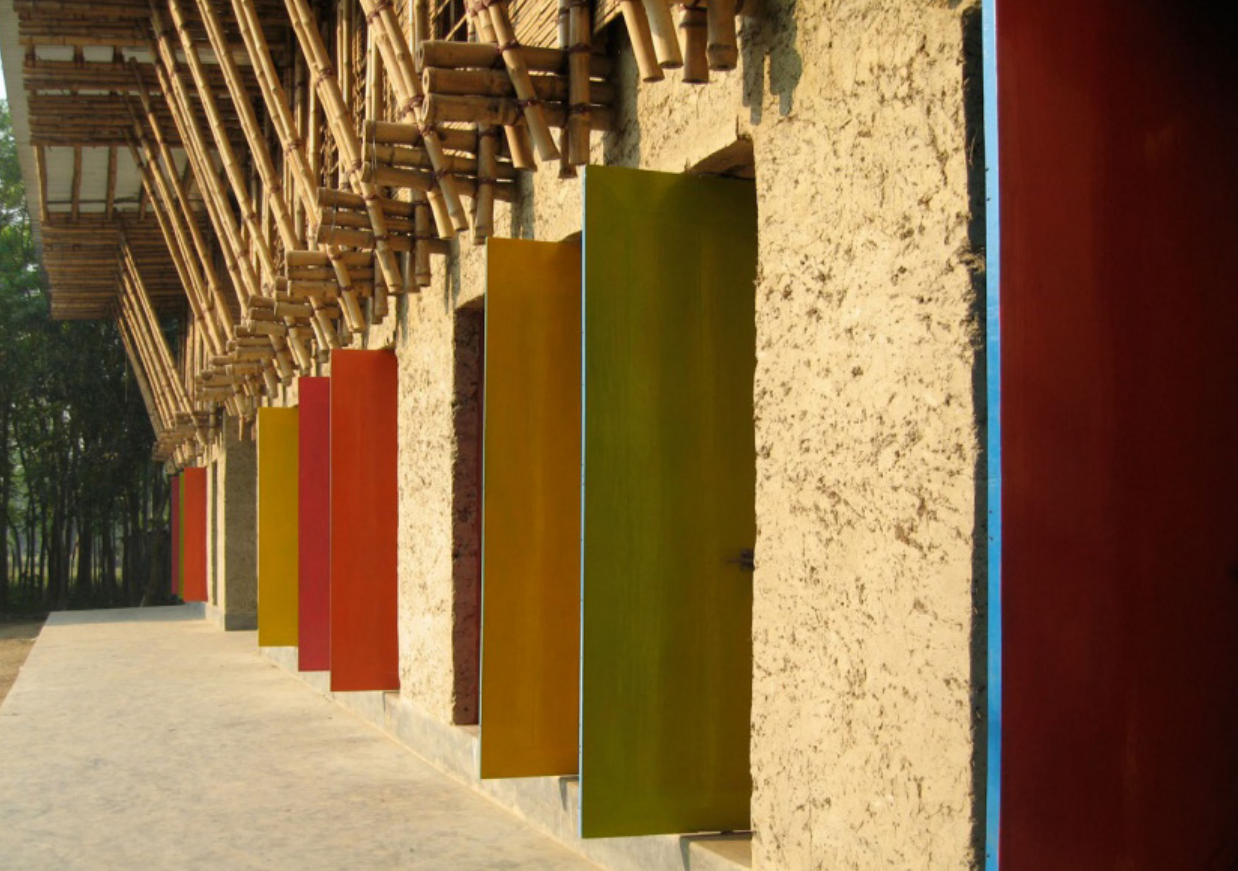
Figure 73 : Façade Hand made school / Photographie : © Kurt Hoerbst
