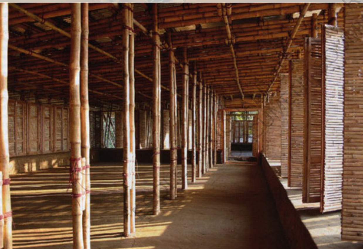
Figure 76 : Etage Hand made school / Photographie : © Kurt Hoerbst
