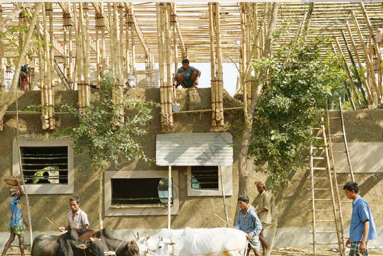
Figure 74 : Façade Hand made school / Photographie : © Kurt Hoerbst
