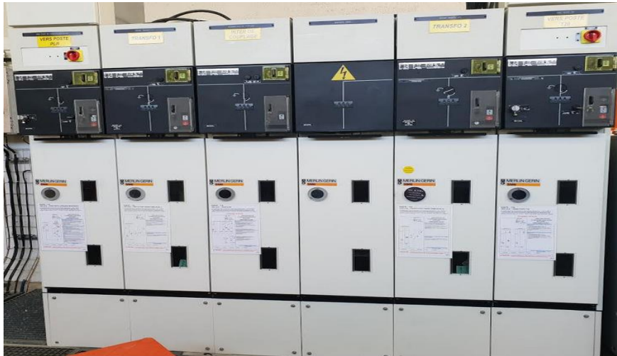
Figure III.1 : cellules SM6-24.
