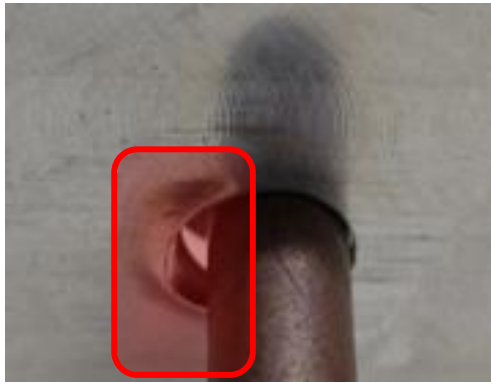
Figure 51 –Matage de fixation.
